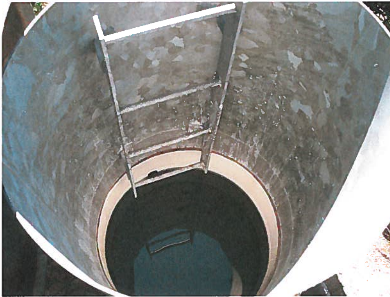
Figure 5: Looking down hatch of 15,000 gallon storage tank
