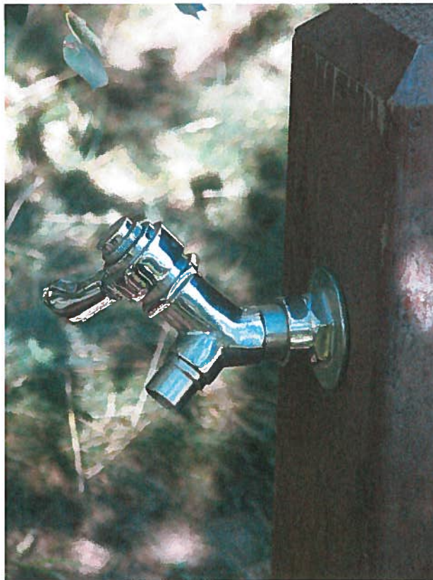
Figure 6: Threadless spigot at campground
