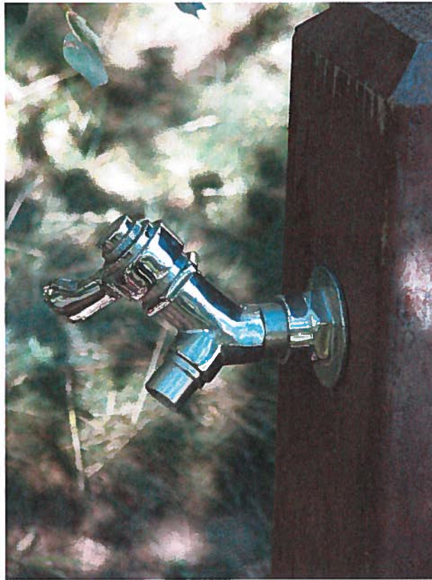
Figure 5: Threadless spigot
