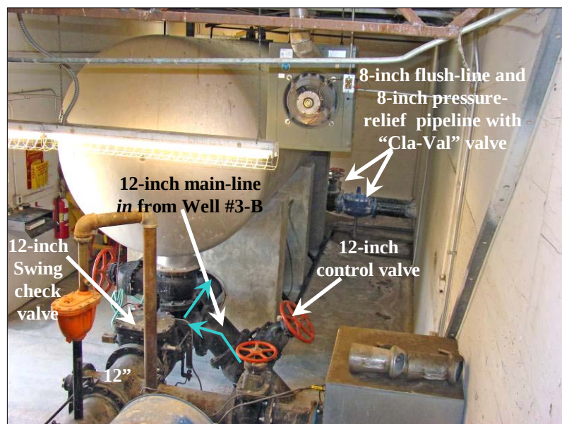
Figure 5. Existing pump house plumbing configuration inside the ISCI Well #3-A pump/control house. The existing plumbing facilities will be used for the new Well #3-B until planned modifications (underway) are completed.
