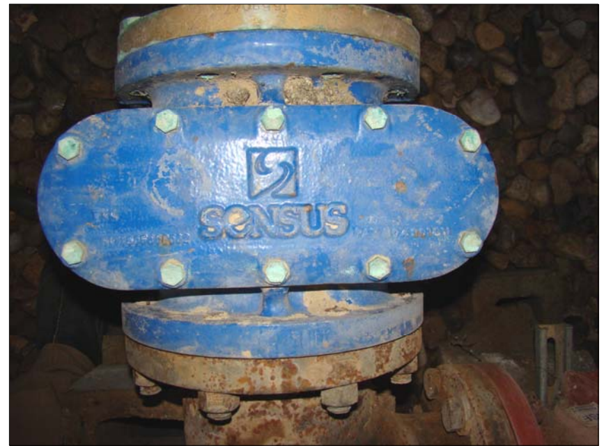
Integral flow-straightener on Sensus Model #W-2000 flow meter of ISCI Well #8.
