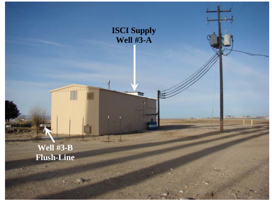
Photo looking west at Well #3-A pumphouse.
