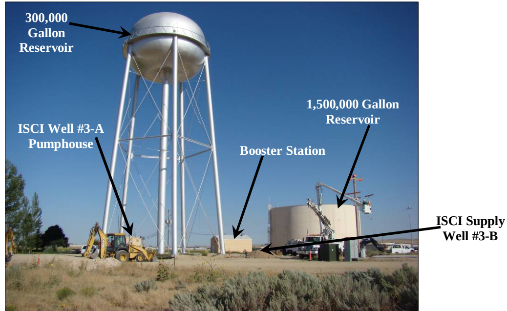
View looking northwest at the ISCI Wells #3-A and #3-B well site.
