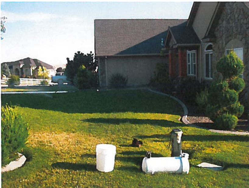
Well with house & front lawn. Fertilizer tank next to well. Tank hooks into sprinkler system at box next to well.
