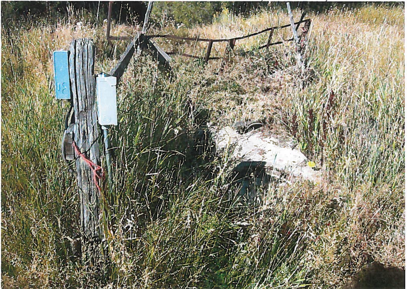
Pump and cistern at lip of canyon
