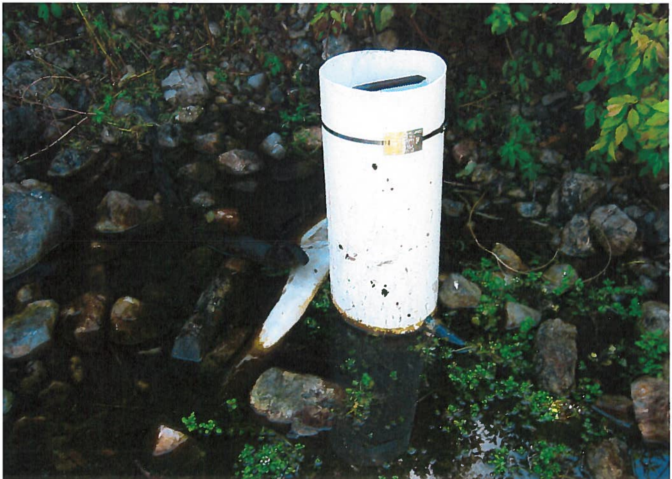
Gunnell - POD and Valve box
