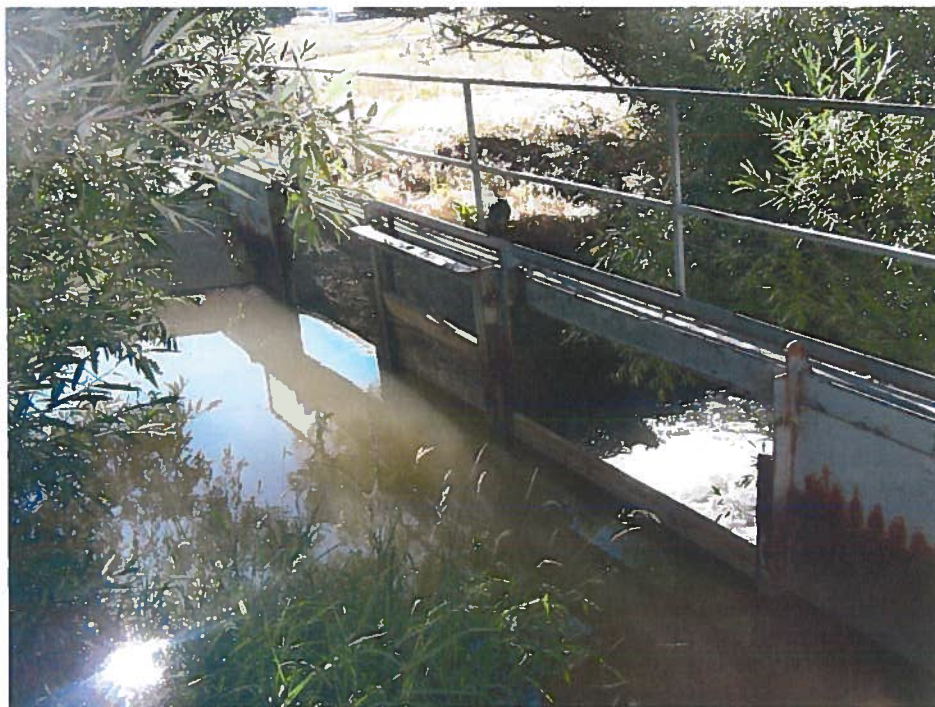
63-12304 License Exam 7/15/2010: Downstream weir/check on Willow Creek facing southeast (downstream).
