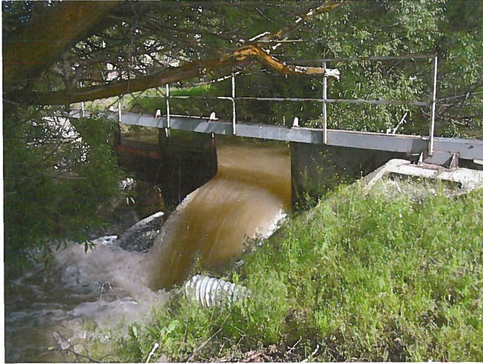
63-12304 License Exam 6/8/2010: Downstream weir/check on Willow Creek facing northwest (upstream). Note large drop on weir between upstream and downstream surfaces.
