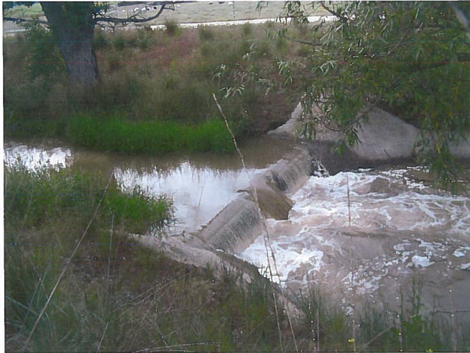
63-12304 License Exam 6/8/2010: Upstream weir on Willow Creek facing southeast. Note vegetation on sides of creek upstream of weir.
