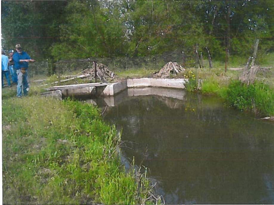
63-12304 License Exam 6/8/2010: Siphon where water is backed up into Middleton Mill Ditch Co and piped under Willow Creek into Canyon Hill Ditch facing west. Culvert that water backs up into Middleton Mill Ditch (P/D) located where Alan Funkhauser (Drainage Dist #2) is standing.
