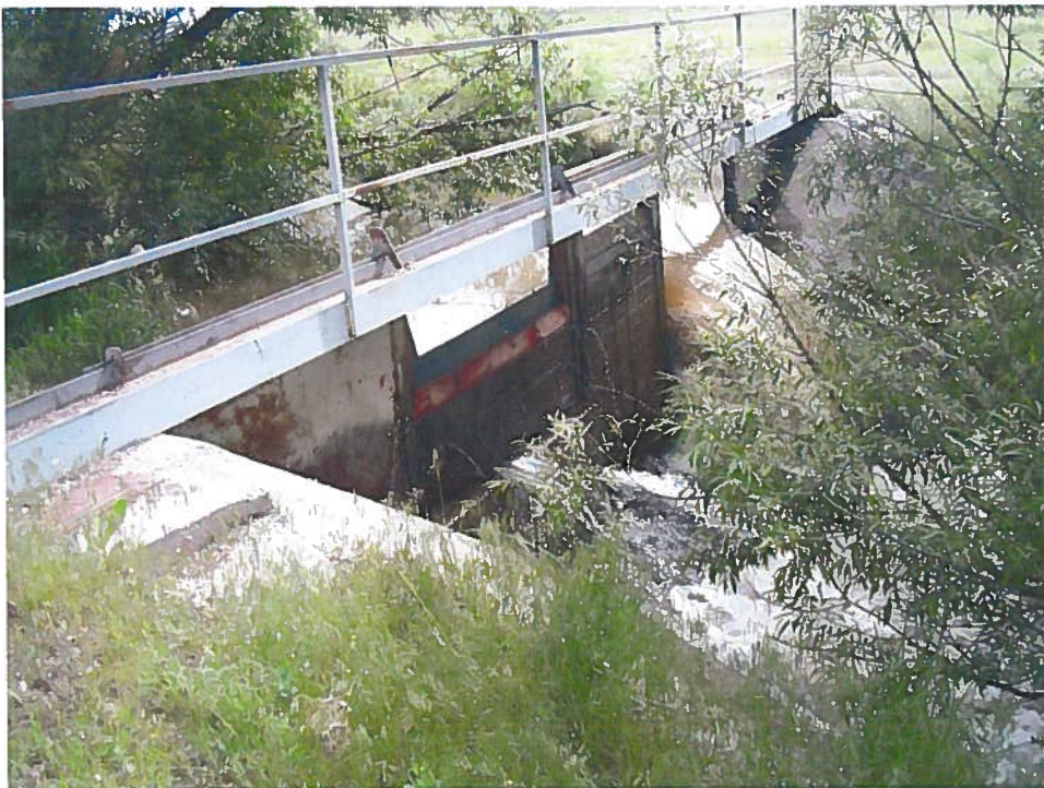
63-12304 License Exam 6/8/2010: Downstream weir/check on Willow Creek facing northeast (upstream).
