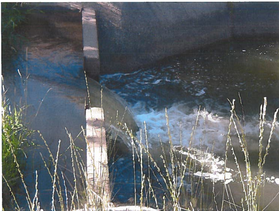
63-12304 License Exam 7/15/2010: Upstream weir on Willow Creek facing south/southeast.
