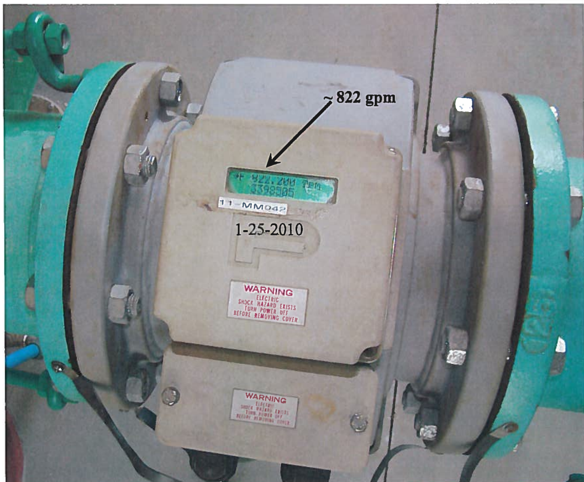
Figure 6. January 21, 2010 photographs of the Kuna Danskin Well #1 flow-meter's digital readout showing 822 gallons per minute at a line pressure of 79 psi during the proof of beneficial use field examination. Line pressure measured with a brace of high-quality gages supplied by Hydro Logic, Inc.
