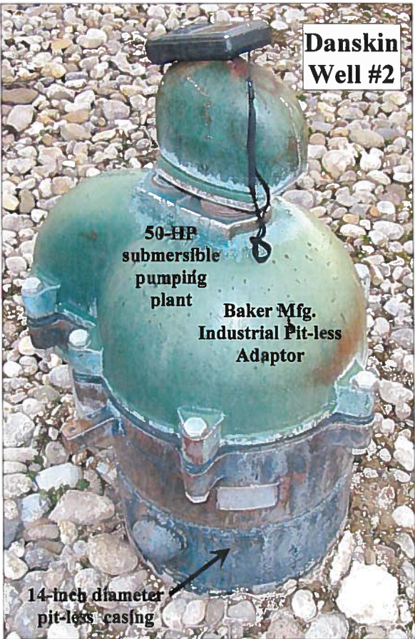
Figure 5. Photos of the Well Heads and Discharge Piping for Kuna City Danskin Supply Wells
