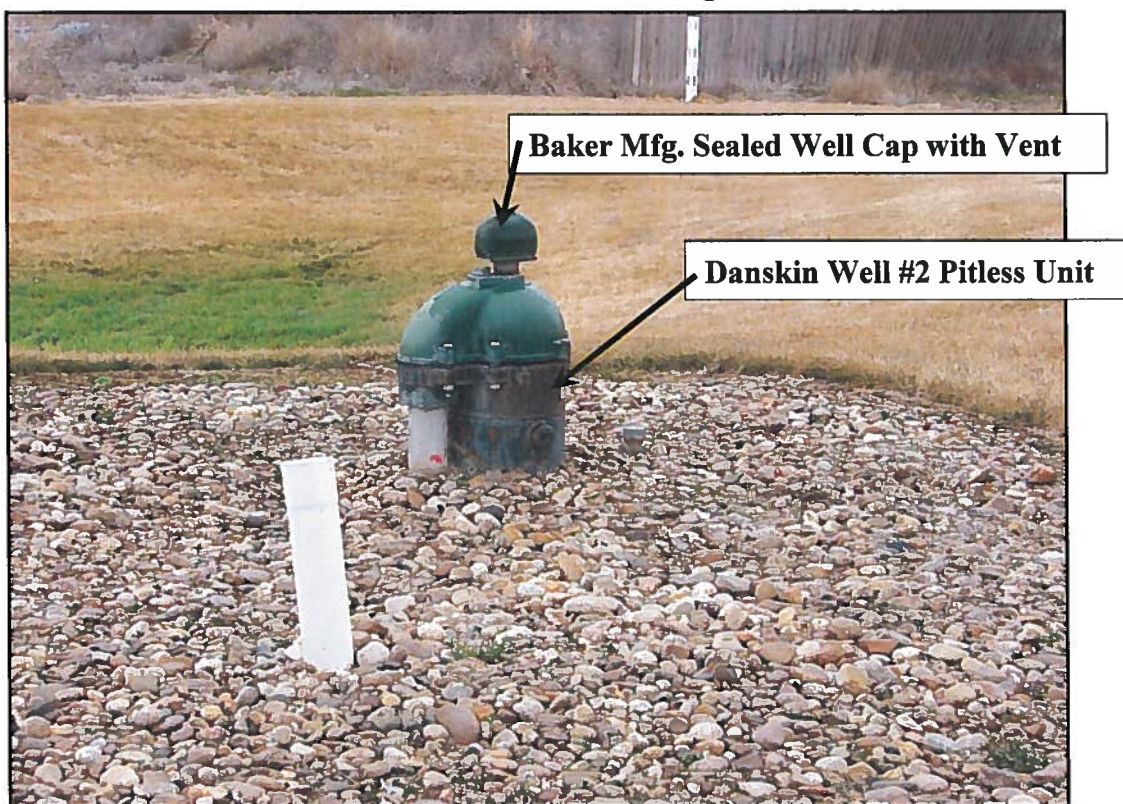
Figure 14. Photos of Danskin Well #2 Pitless Unit and Measuring Tubes
