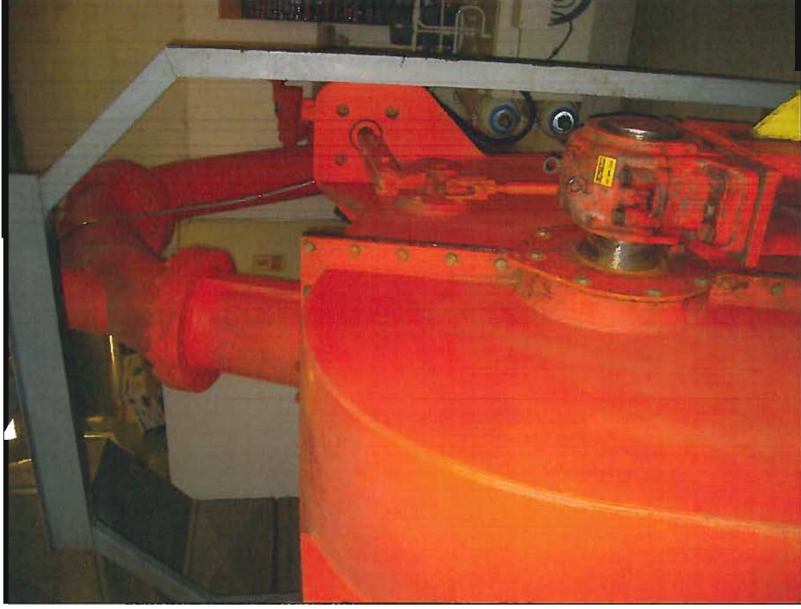
Picture 15 – turbine in foreground. Behind and above turbine the upper leg or line of the penstock can be observed.
