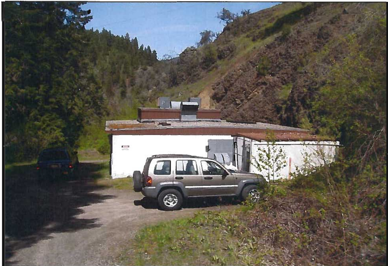
Picture 11 – photo of east face of power house. The buried penstock runs almost directly under the middle of the car observed in the foreground.
