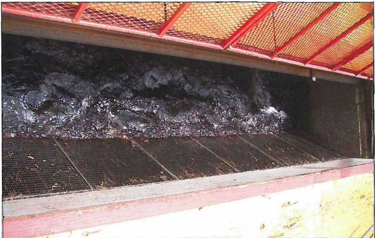
Picture 4 – photo of upstream screen at penstock intake.
