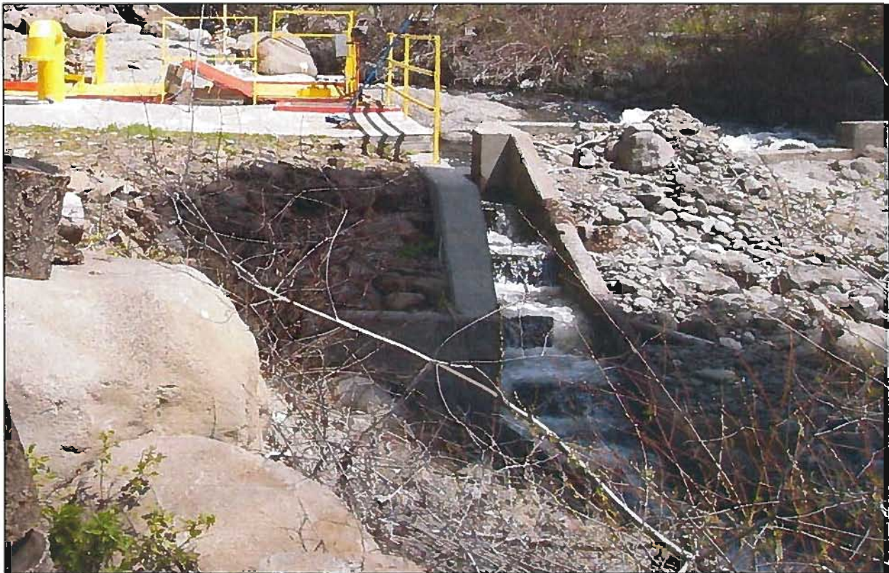
Picture 6 – photo of fish passage ladder taken from below (downstream) of the ladder.
