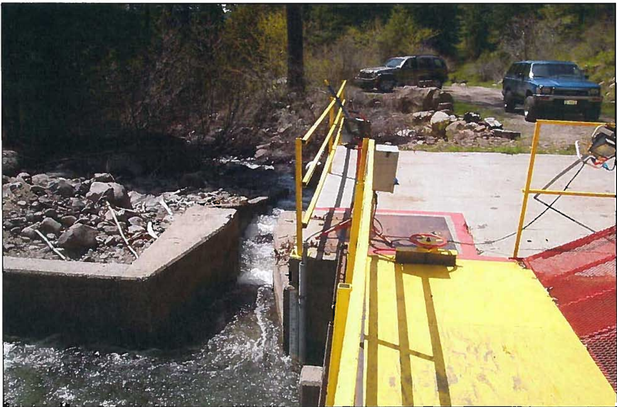
Picture 5 – photo of inlet to fish passage channel. Note Parshall flume built into the passage and staff gage and stilling well (houses pressure transducer) on the right face of the entrance.
