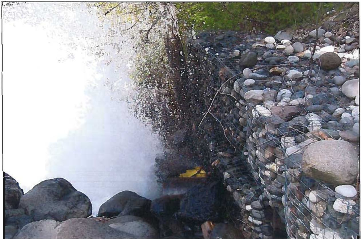
Picture 25 – discharge of water back to Elk Creek – side view.
