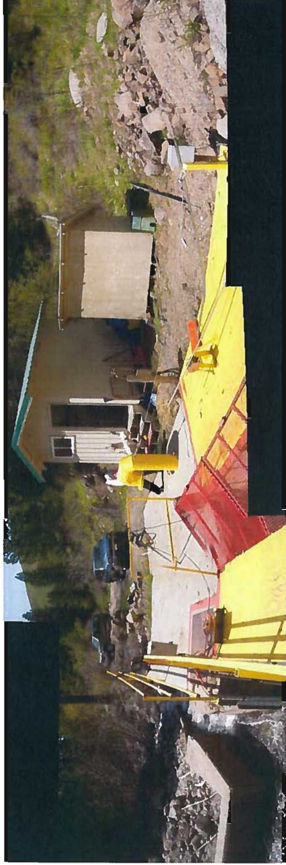
Picture 1- Panoramic photograph of intake works including diversion dam (left), fish flow by-pass channel (middle), and intake works (right).
