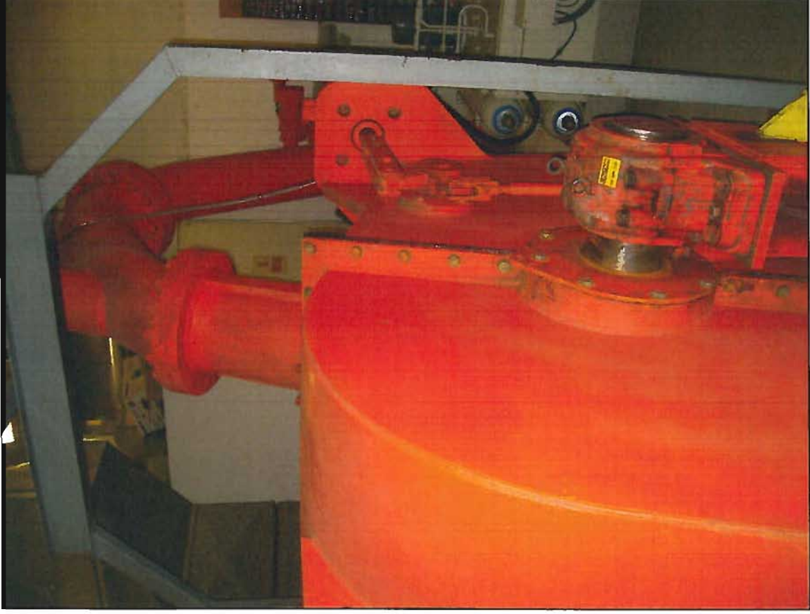
Picture 15 – turbine in foreground. Behind and above turbine the upper leg or line of the penstock can be observed.
