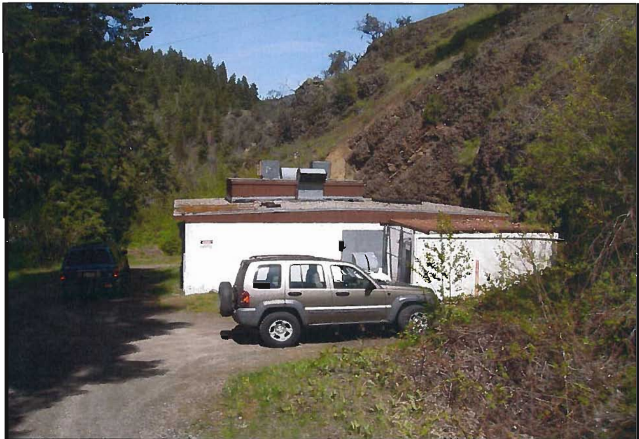
Picture 11 – photo of east face of power house. The buried penstock runs almost directly under the middle of the car observed in the foreground.
