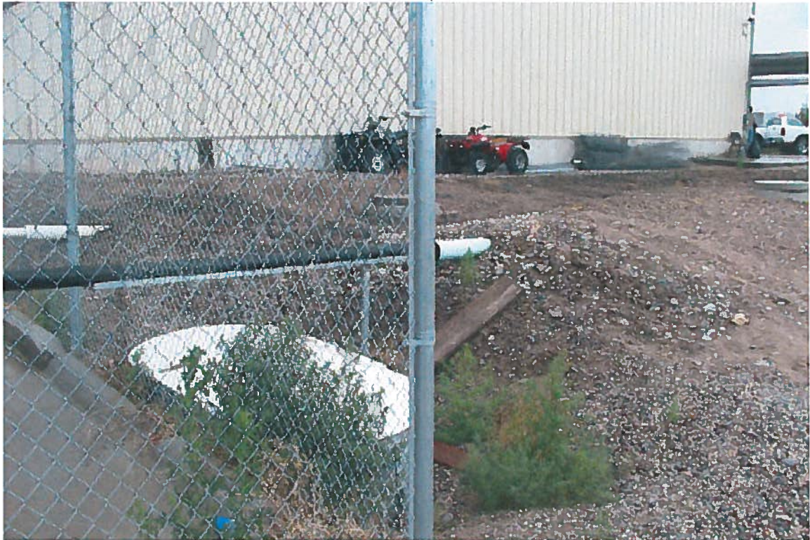
Wastewater pipe enters ground
