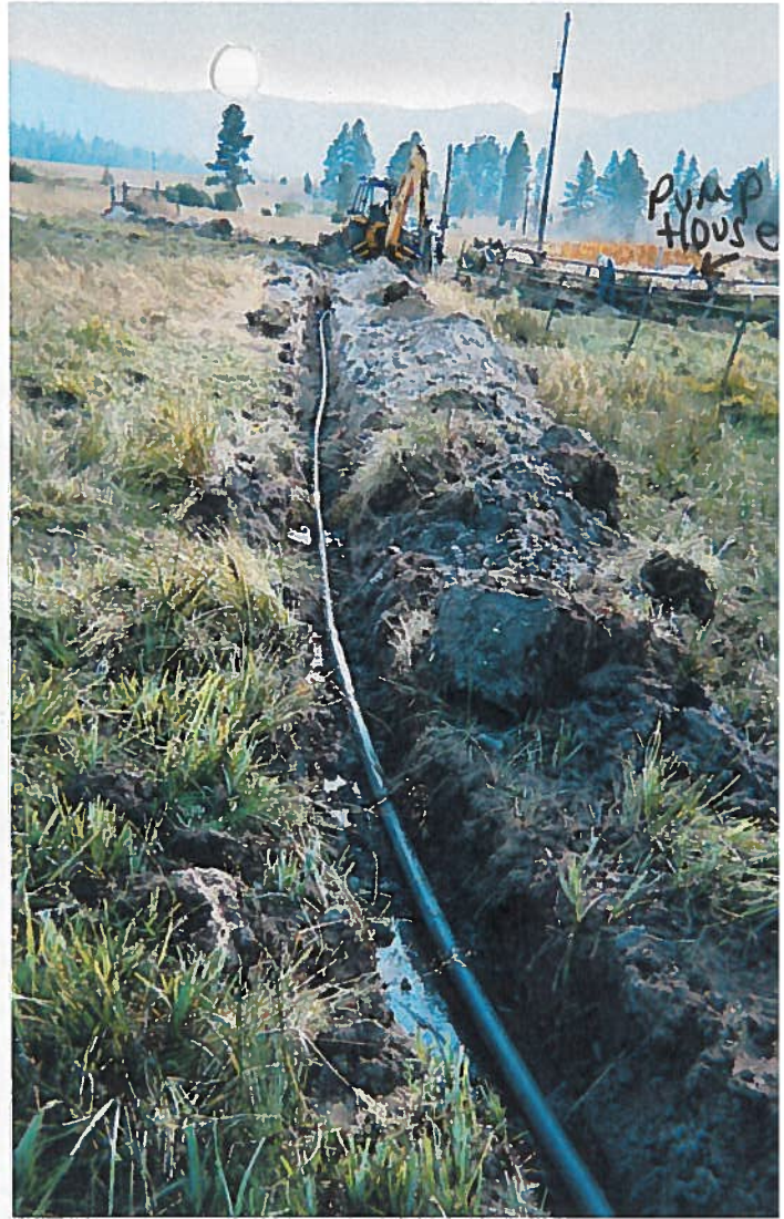
2" pipe From Macgregor's to Pancheris
