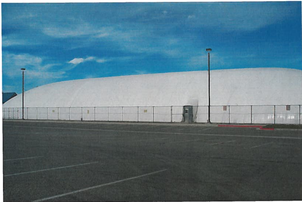
City Pool Building Looking NW From SE Corner
