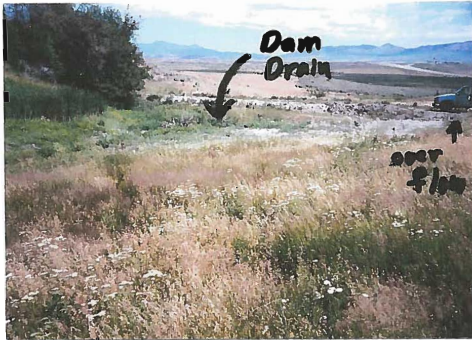
looking North at Dam - showing drain and over flow locations -
