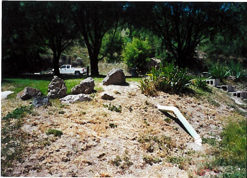
Downstream collection box with overflow pipe to river. Permit # 29-7936
