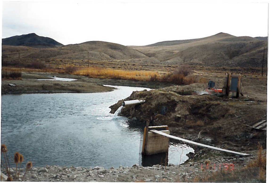
Raceway Out Flow Entering Settling Pond On Warm Creek Looking Upstream
