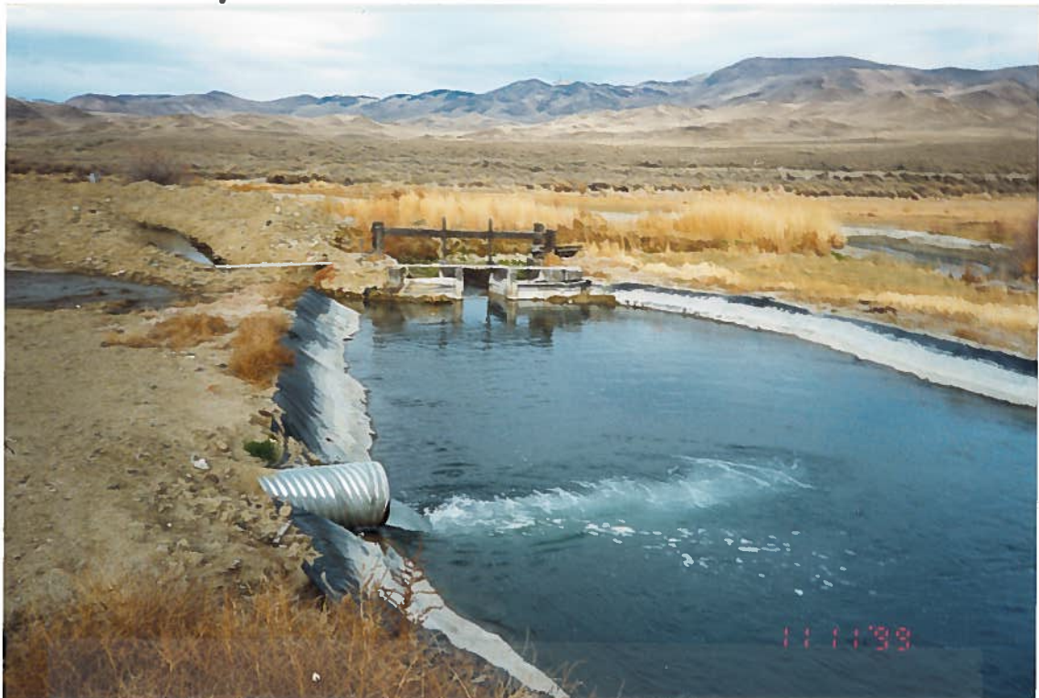
Outflow From Ep. Aq. Raceways Entering Ingram Pond For Settling
