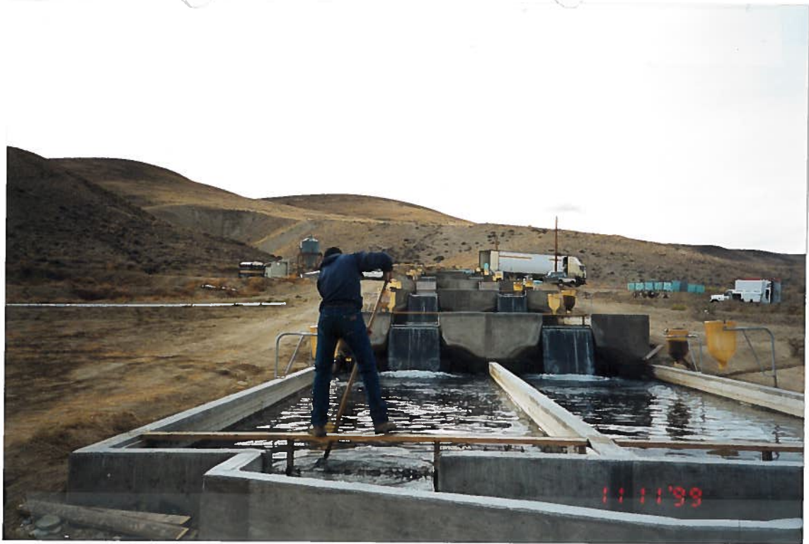
Lower Raceways Looking Upstream Towards Canal
