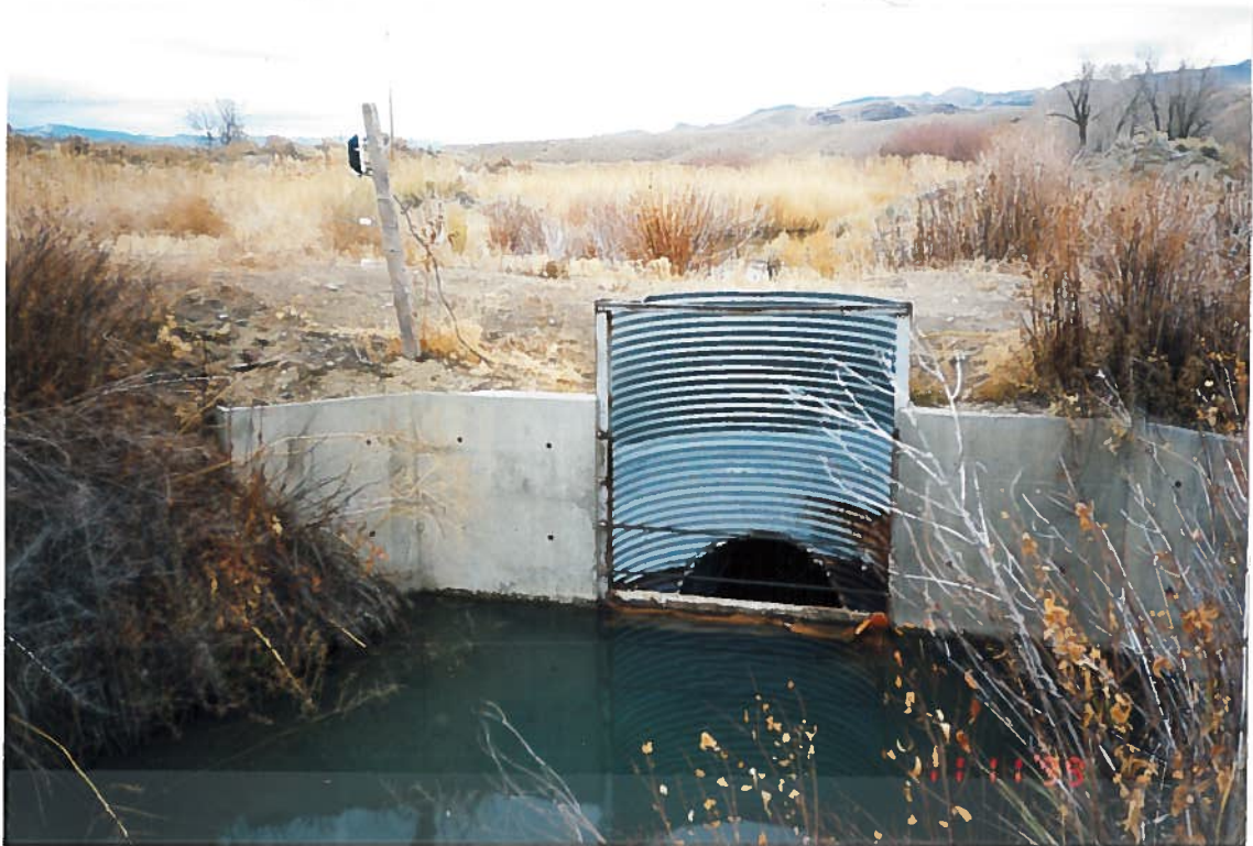
Controlling Works On Warm Springs Canal
