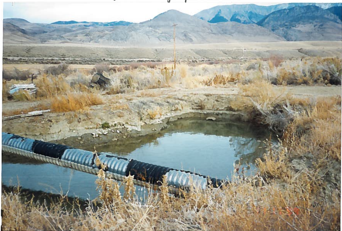
Inlet From Warm Creek Ditch; Pipeline From Brood Ponds
