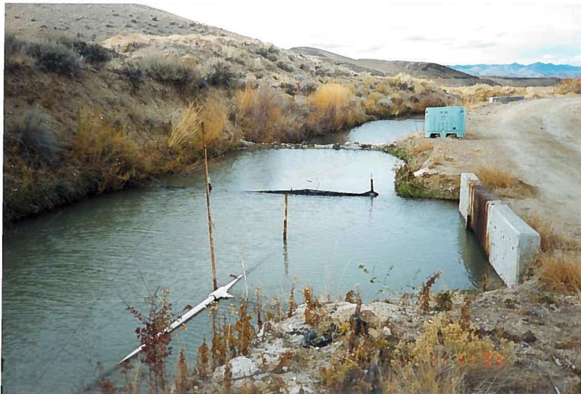
Warm Springs Canal; Inlet + Outlet For Raceways (Looking Downstream)
