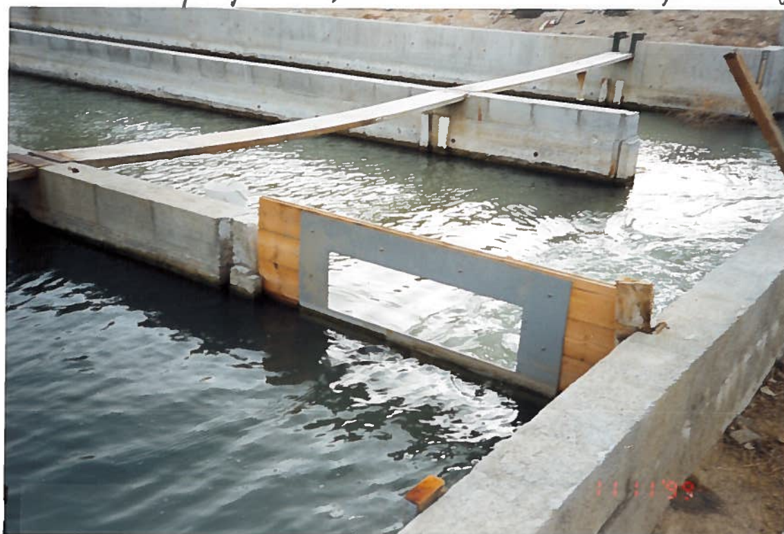
Measuring Device Above Outlet (Actual Orifice Is Underwater)
