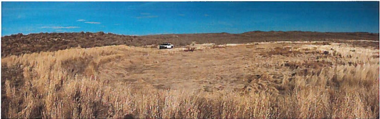
Figure 2: View from South side of NENW reservoir looking northeast.
