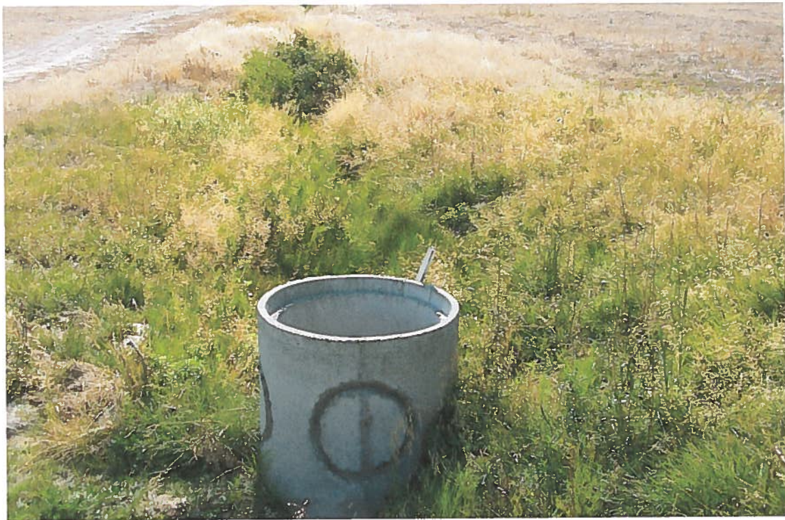
Figure 3. Lunch Creek Pipe Inlet, ditch looking uphill
