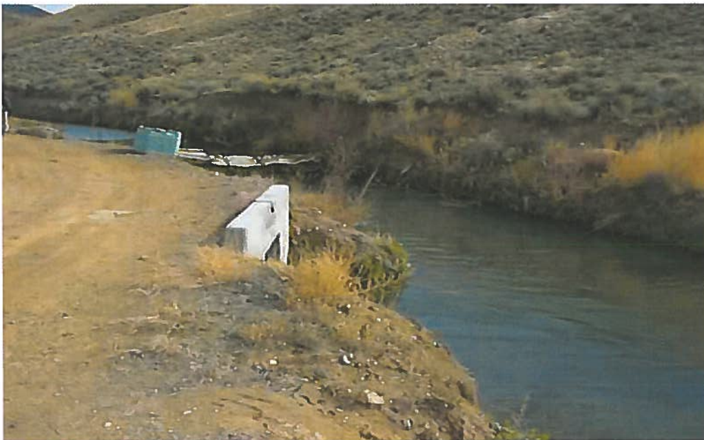
Below: Discharge from hatchery to canal (foreground). Note diversion dam and hatchery intake in background.
