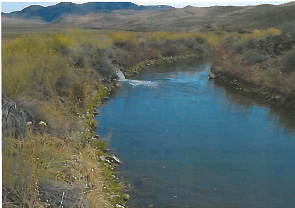
Below: Discharge to canal from Morganroth re-lift pump.
