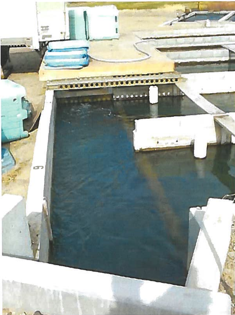
Lupher tailrace and return flow to canal. Note flow from large upper raceways on right side of photo. Submerged orifice located underneath footbridge in middle of photo.
