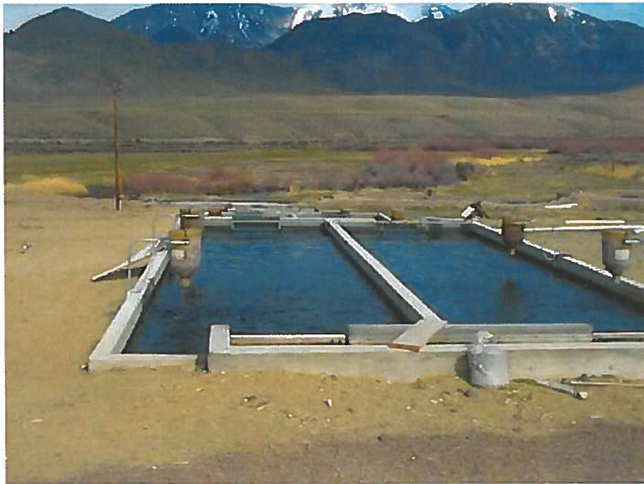
Above: Lupher Hatchery. Lower stair stepped raceways.
