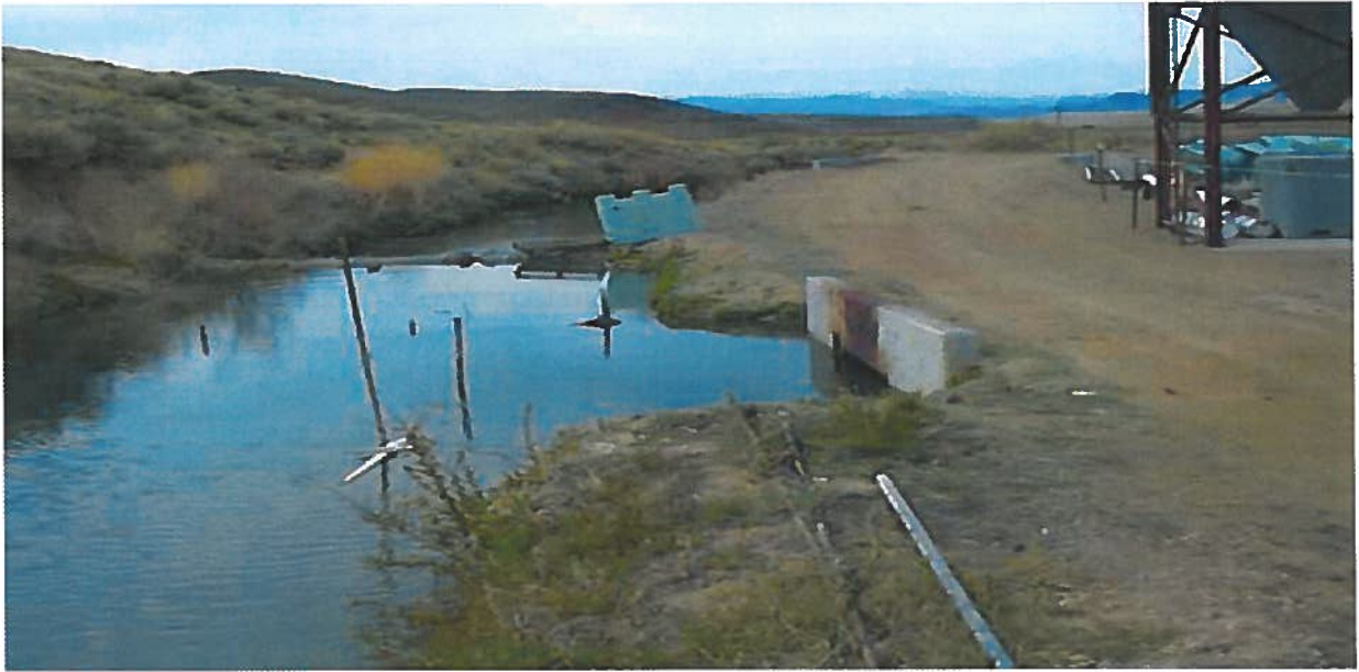
Lupher Hatchery re-diversion from Warm Spring Canal: diversion dam across canal checks water into concrete intake box and channel.
