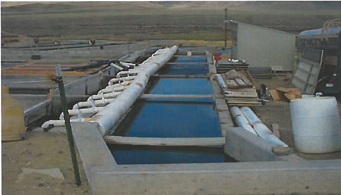
Lupher Hatchery. Upper head-race channel from canal re-diversion. Submerged orifice in channel about halfway down headrace. PVC pipe line returns water to raceways on left from settling pond below lower raceways. Note stair-stepped lower raceways in background.
