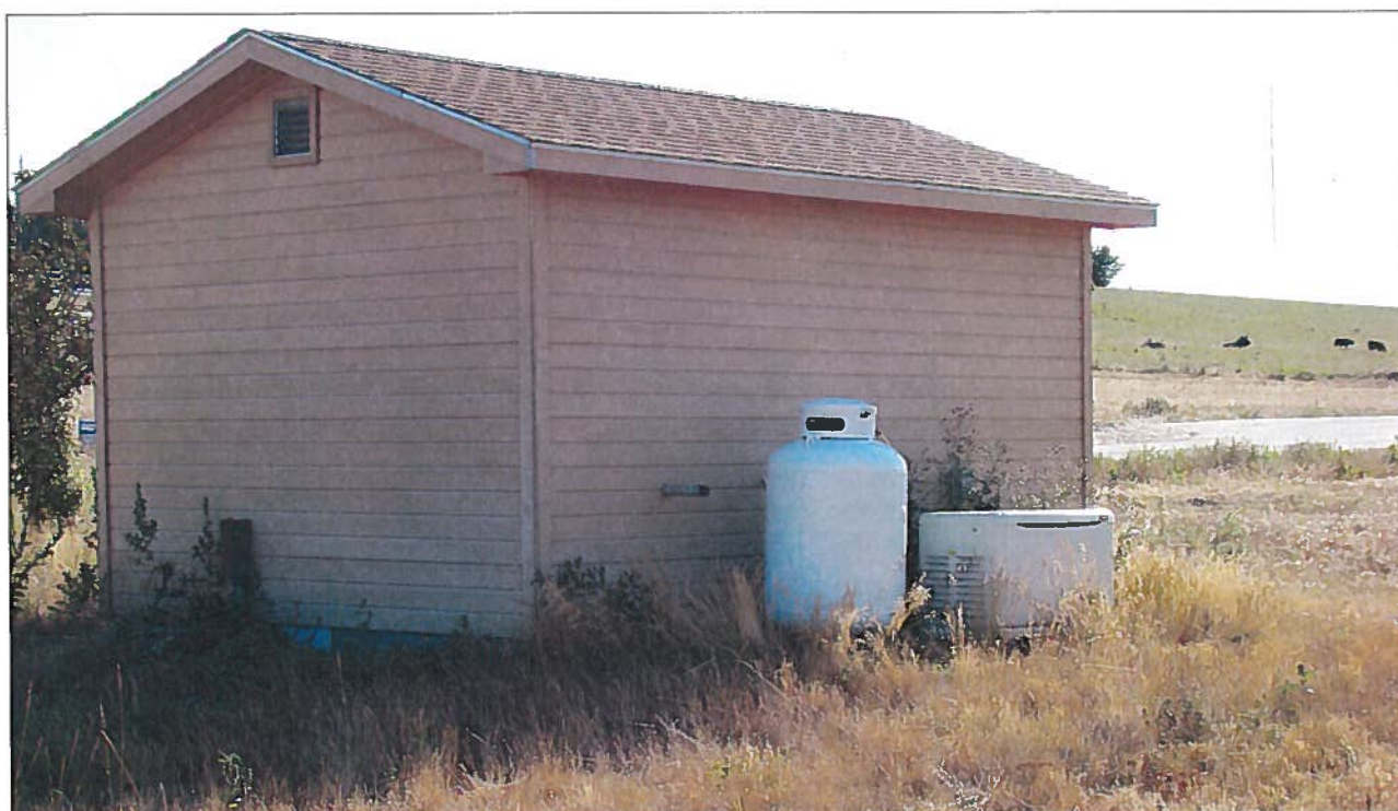
a) July 26, 2011 photograph looking northwest at Well #1 pump house.
