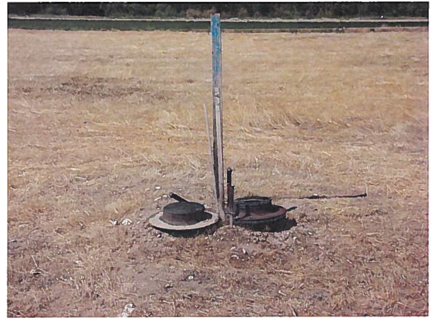
Water utility "stub-ins" for Southshore II subdivision Lots 3 and 4.
