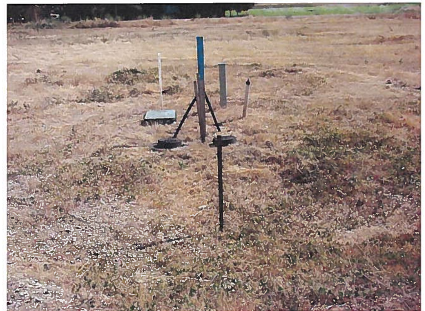
Water utility "stub-ins" for Southshore II subdivision Lots 14 and 15.
