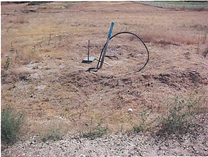
Water utility "stub-ins" for Southshore II subdivision Lot 9.
