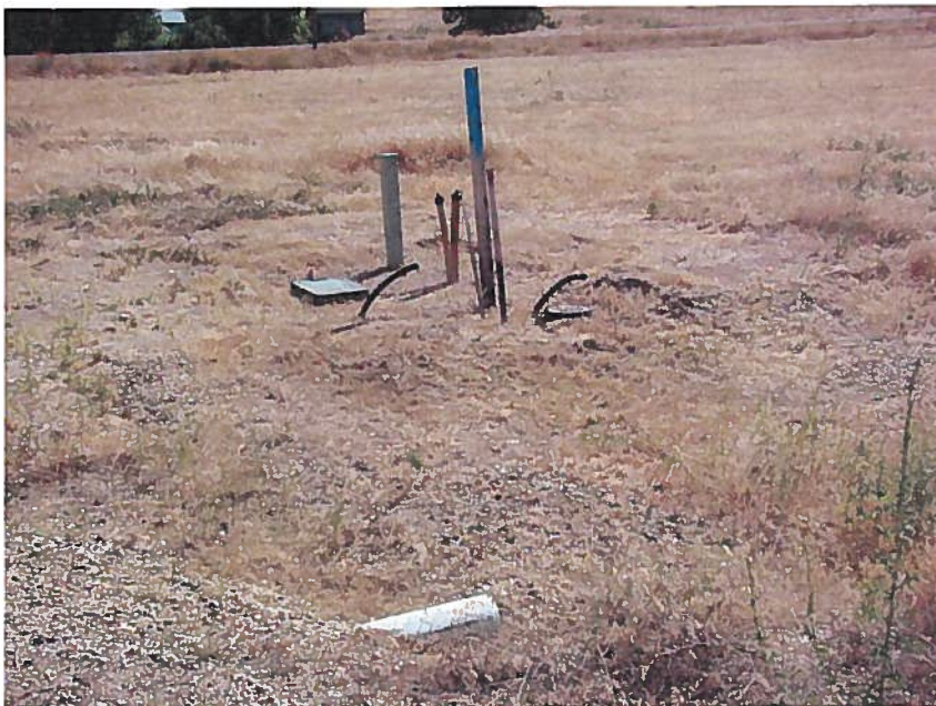
Water utility "stub-ins" for Southshore II subdivision Lots 12 and 13.
