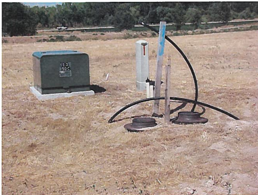
Water utility "stub-ins" for Southshore II subdivision Lots 5 and 6.
