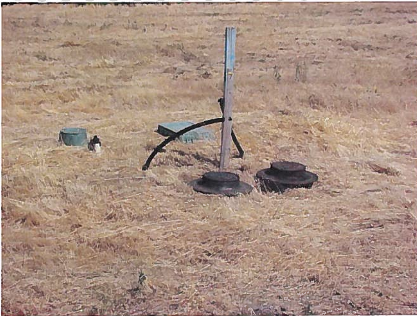
Water utility "stub-ins" for Southshore II subdivision Lots 1 and 2.
