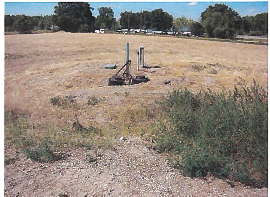
Water utility "stub-ins" for Southshore II subdivision Lots 7 and 8.
