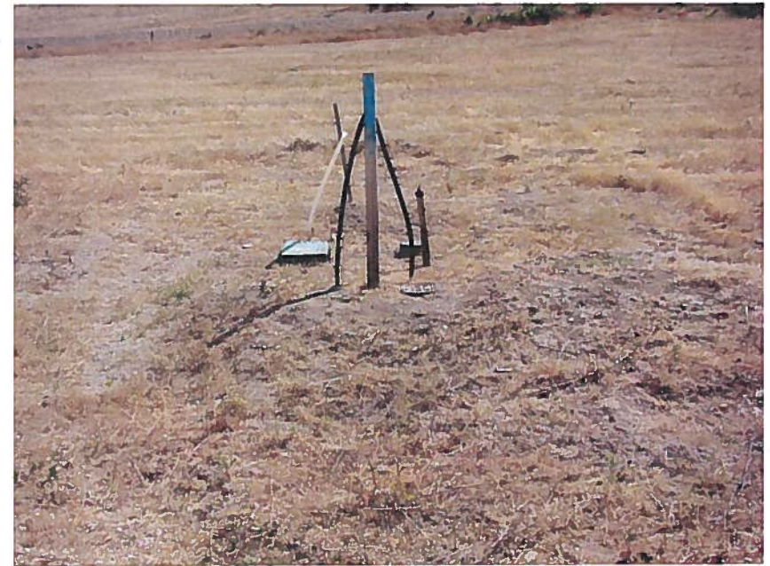
Water utility "stub-ins" for Southshore II subdivision Lots 10 and 11.
