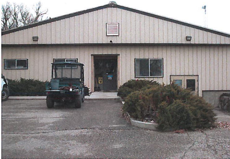
Figure 3: Front Entrance to Wet Labs
