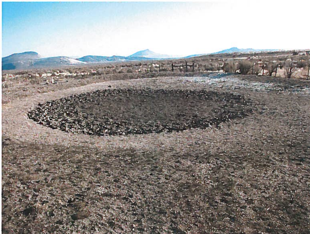
Figure 2: Reservoir from ground level looking northeast 11/15/2011
