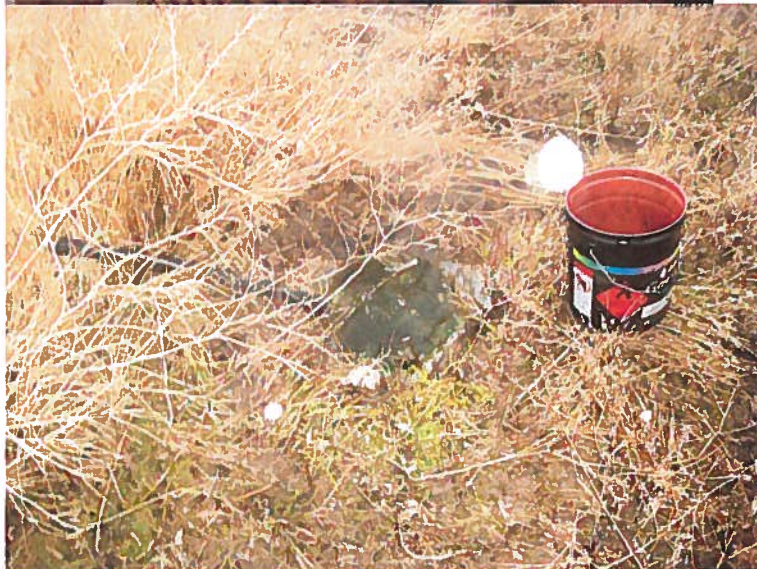
Discharge point from shop/guest house.
