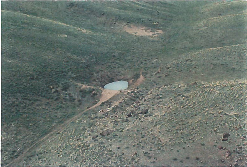
Figure 1: Aerial photo of Curve Reservoir
