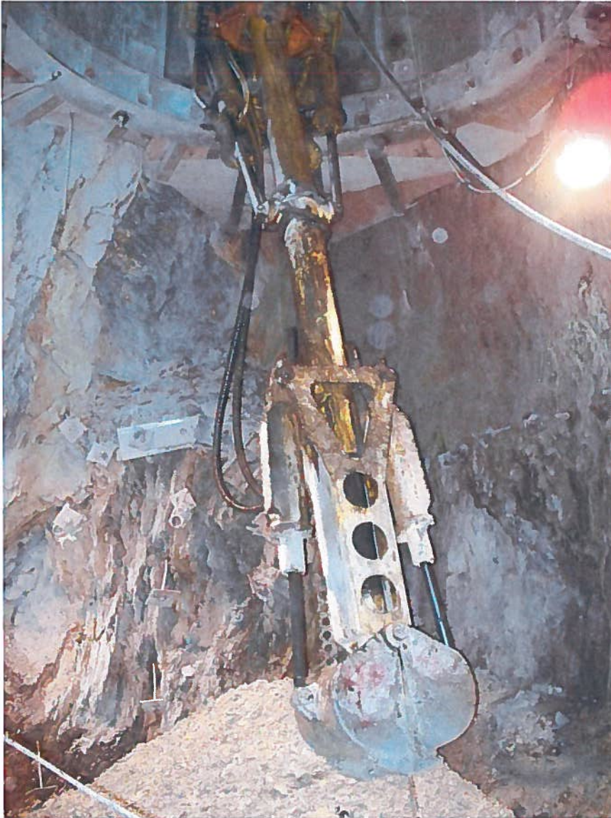
Figure 4. U.S. Silver's Galena Shaft repair, showing Cryderman mucking machine at work below new concrete linings.
