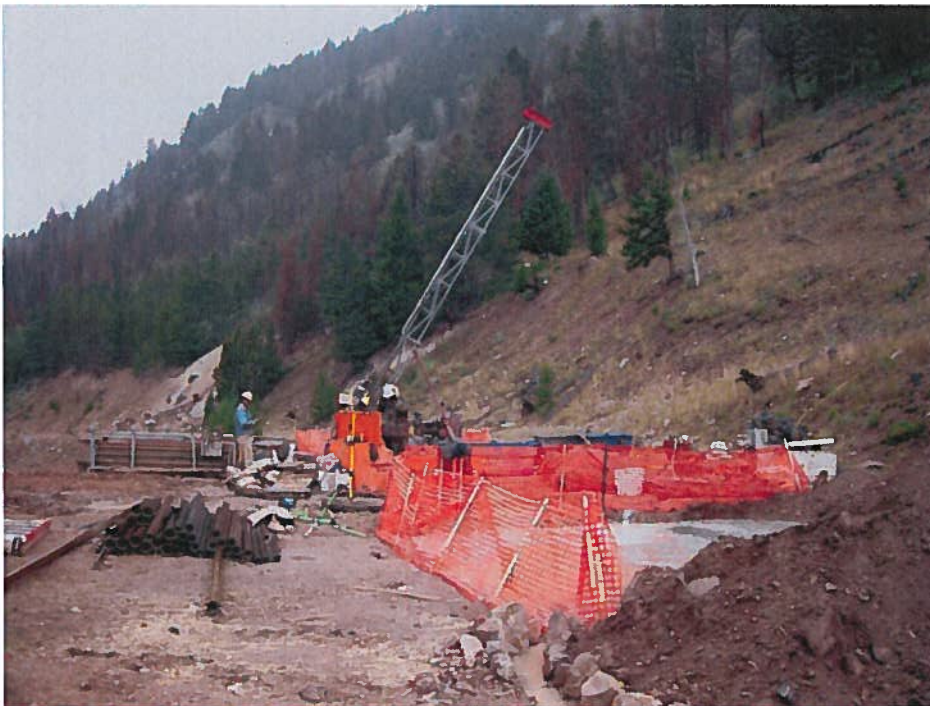
Figure 10. Drilling at Midas Gold's Golden Meadows project, Valley County.
