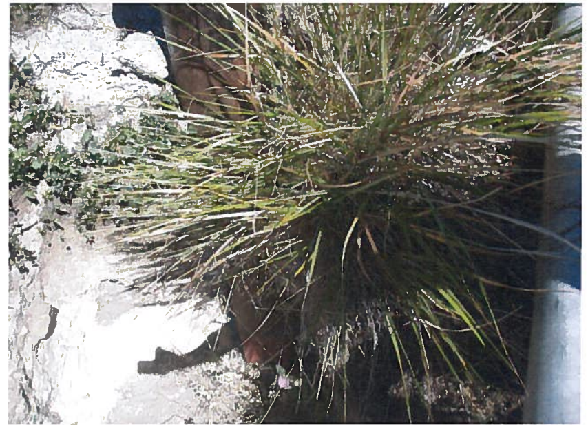
Photo #27 Electrical Connection area & Pitless Adapter
