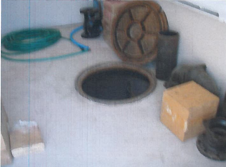
Photo #3 Former Access Hatch to Well #1 Piping & Equipment
