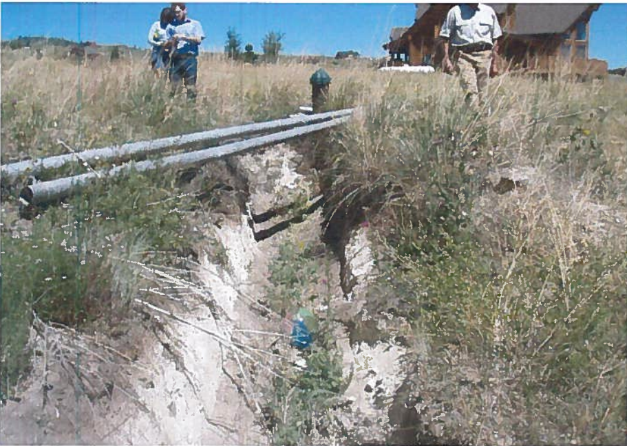
Photo #28 Trench to connect Well #2 in the Future
