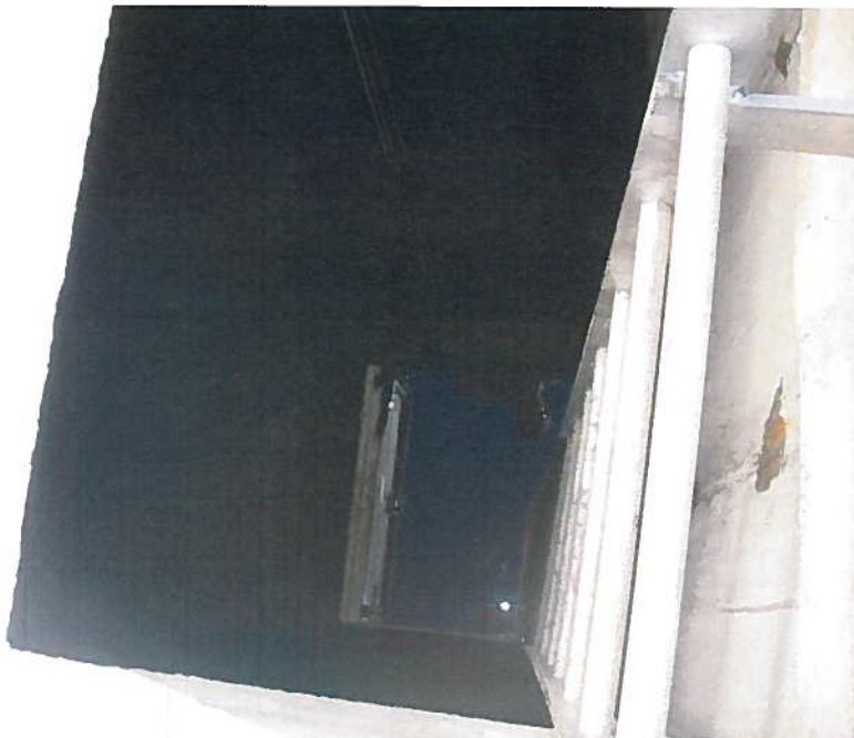
Photo #21 Interior of the Storage Reservoir
