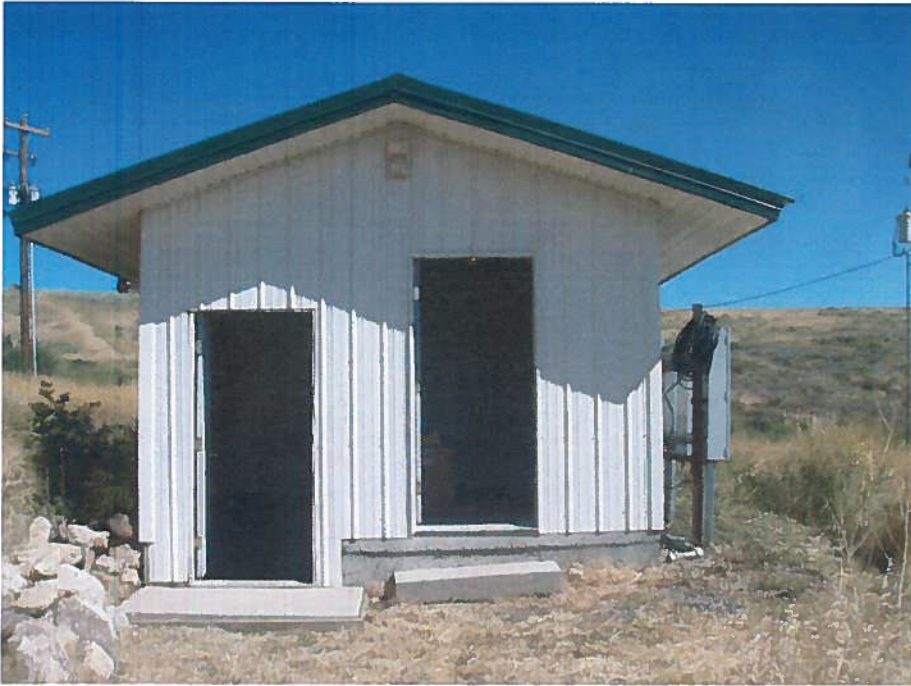
Photo#1 Loveland Well House Well #1
