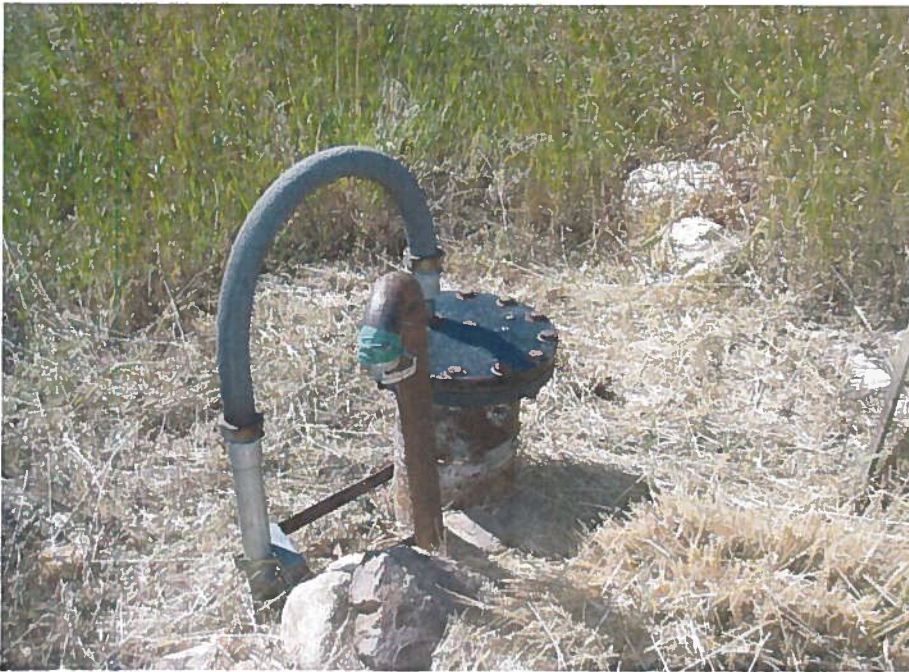
Photo #15 Well #1 With The Vent
