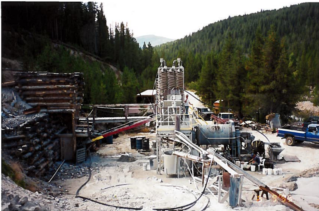
77-7310 Field Exam 9/6/1995 Photo #2: Mill Site (P/U).
