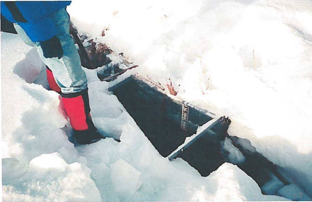
Parshall Flume on Dip Creek at Property Boundary
