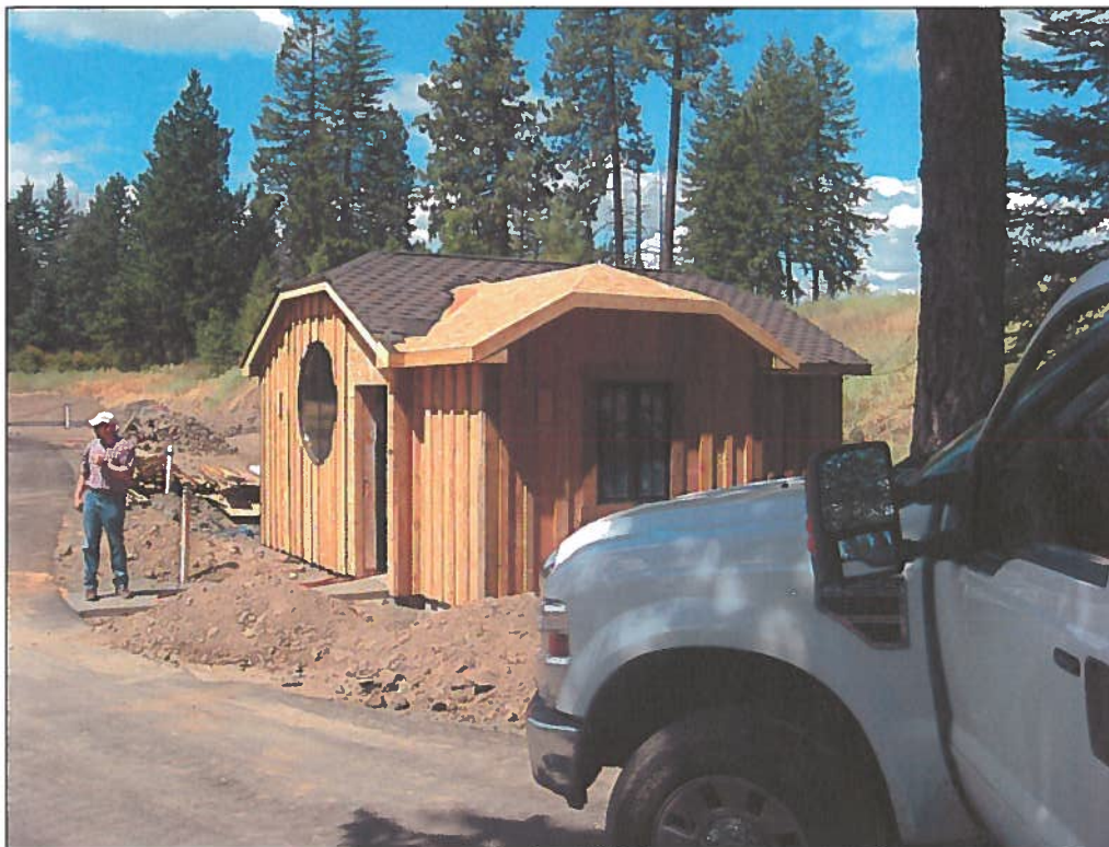
Photo 7: Municipal potable water system booster station.
