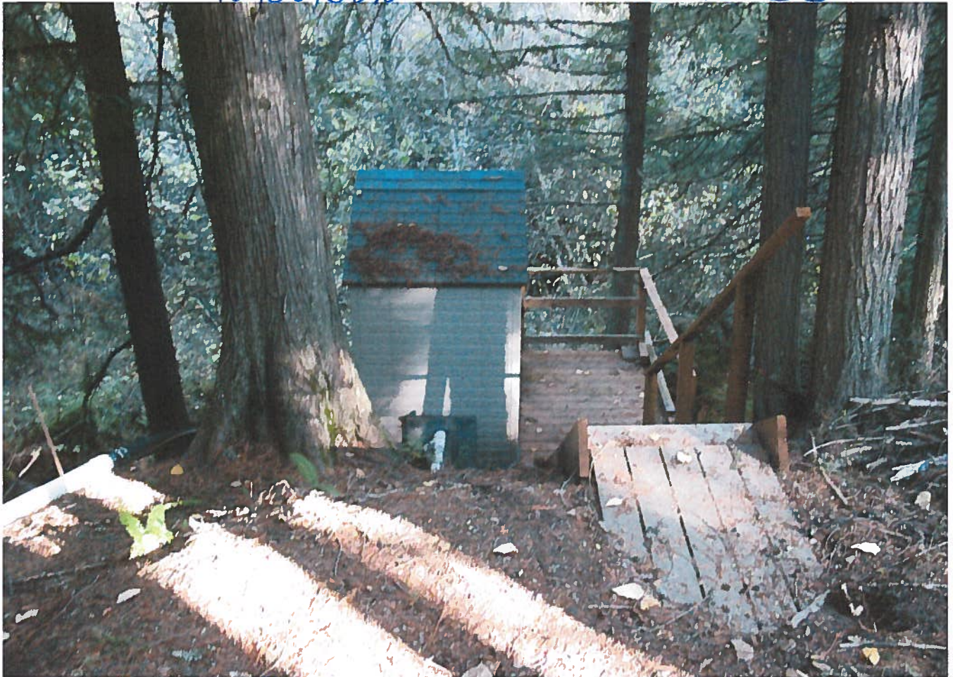
Power Generating House
