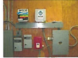
Pump house 1994 Well.JPG
