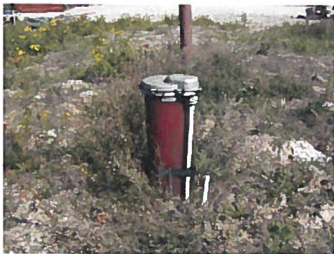
Water tight well cap with screened vent
