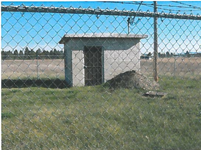
Well No. 2 Building
