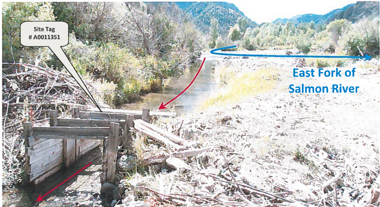
ABOVE: View of point of diversion for 72-167751.
