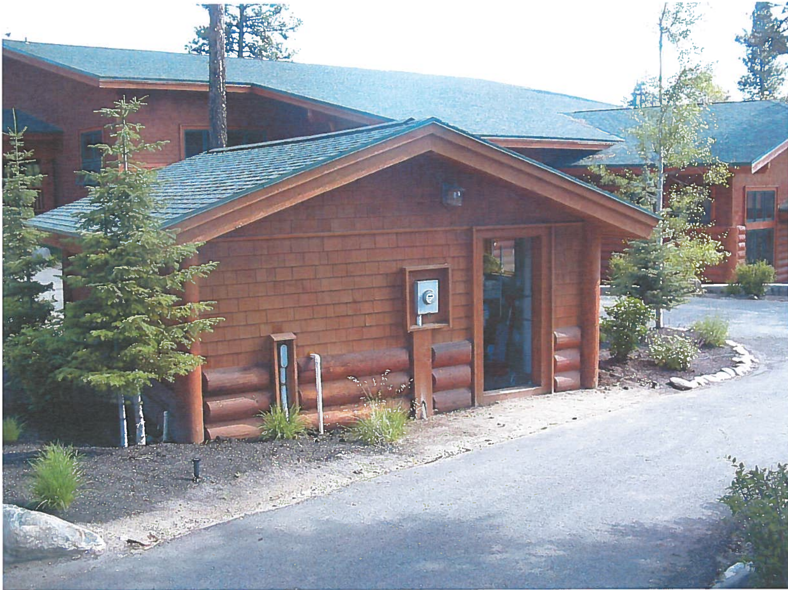
Building with Pump Panel and Piping
