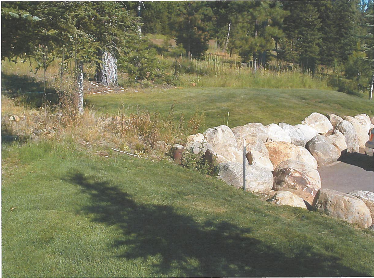
Well No. 1 at Edge of Parking Lot
