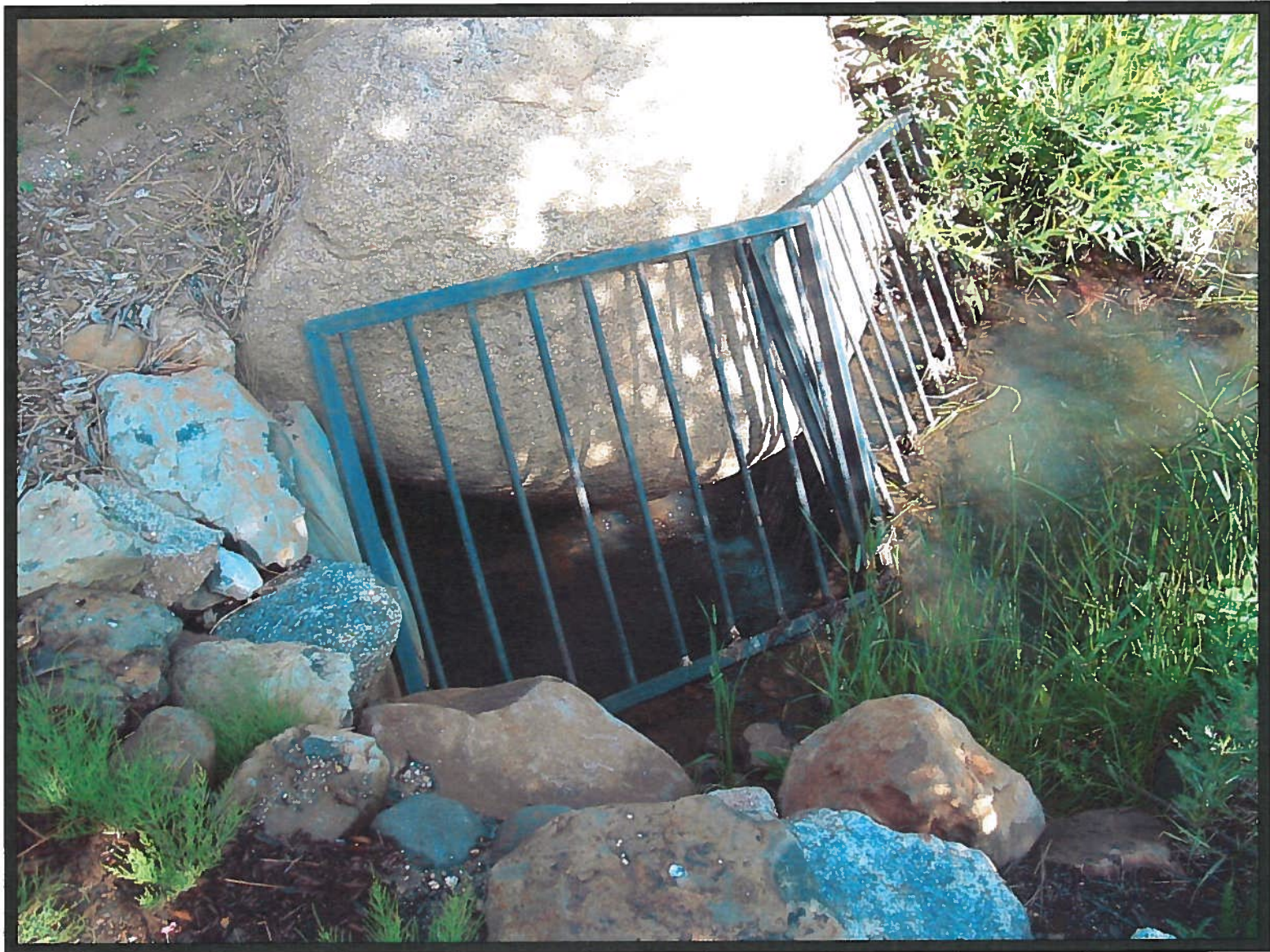
Unnamed Stream Bypass Culvert Inlet
