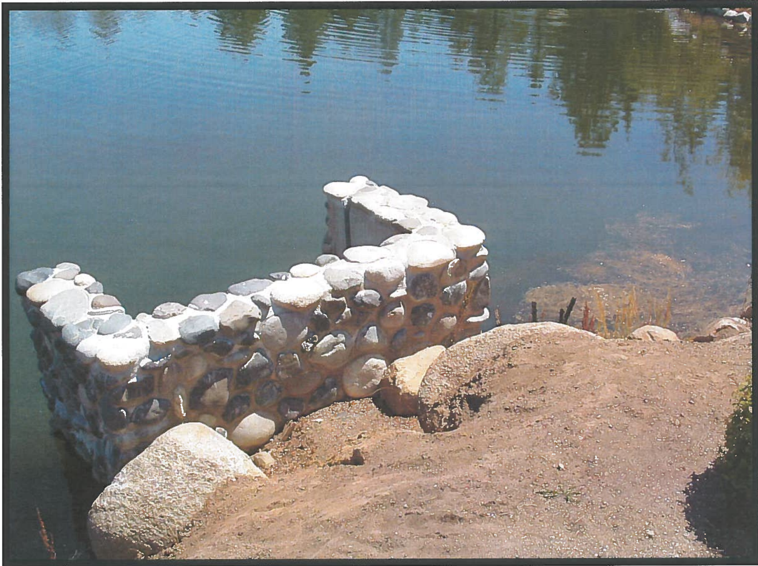
Betsy Pond Overflow to Recirculation Pump
