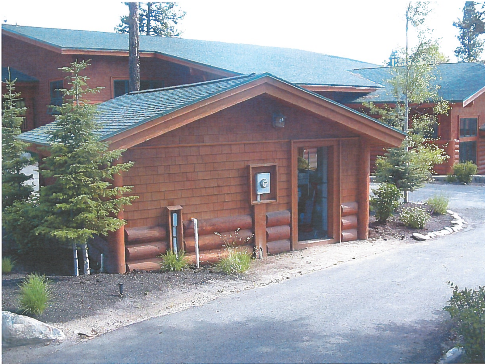
Building with Pump Panel and Piping
