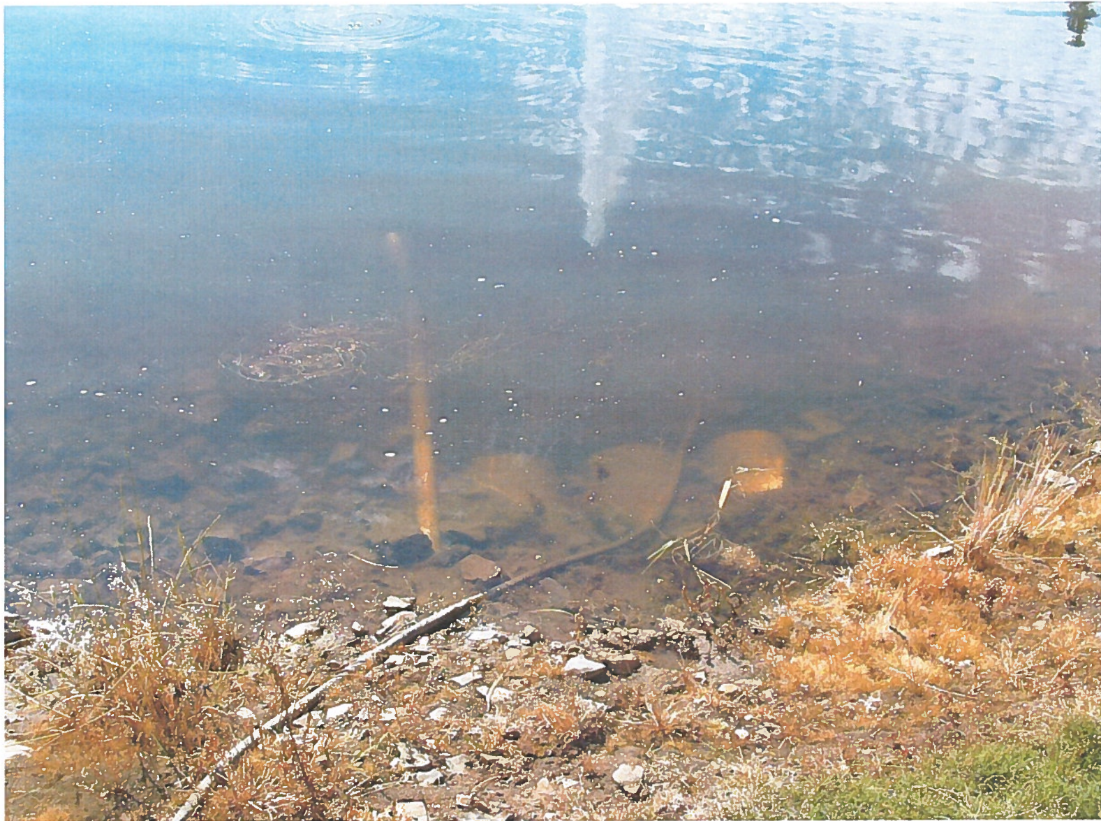
Inlet Pipe from Well 1 at Betsey Pond
