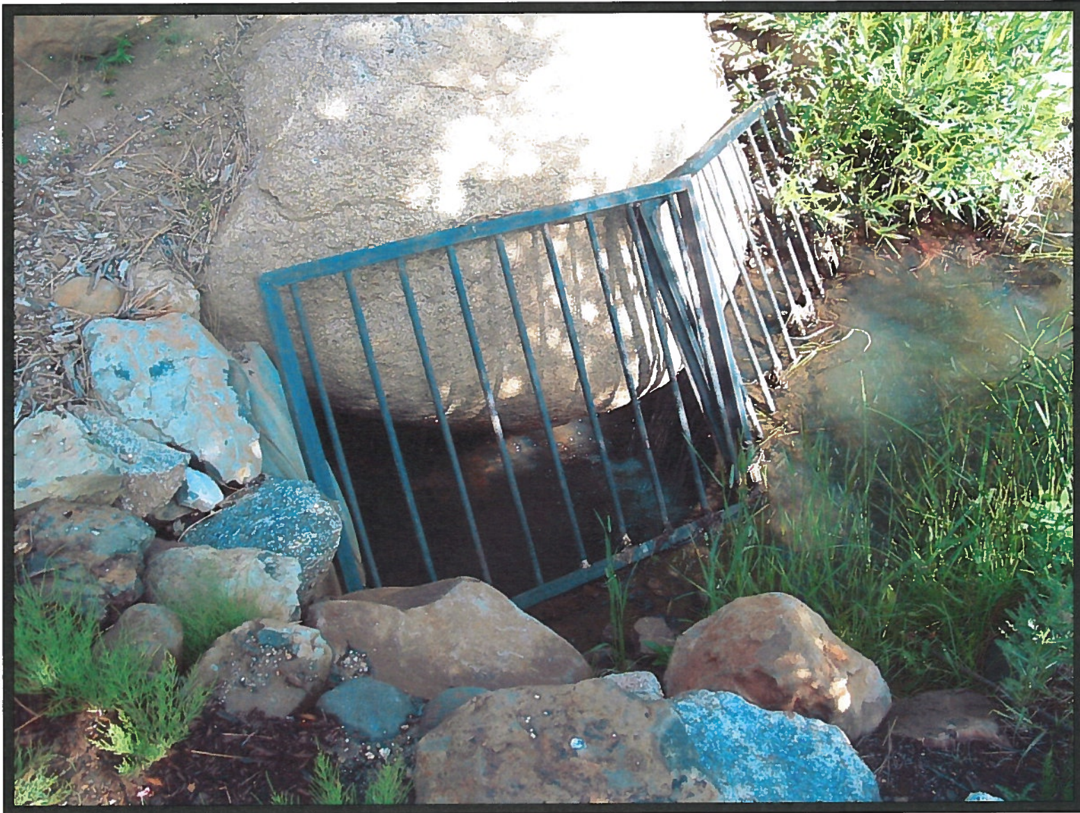
Unnamed Stream Bypass Culvert Inlet
