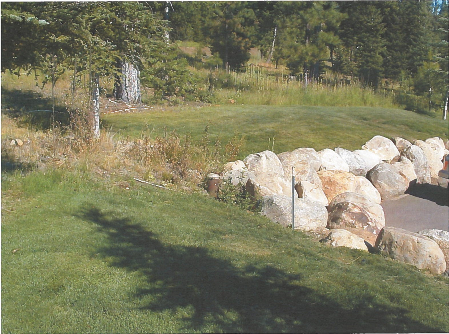
Well No. 1 at Edge of Parking Lot
