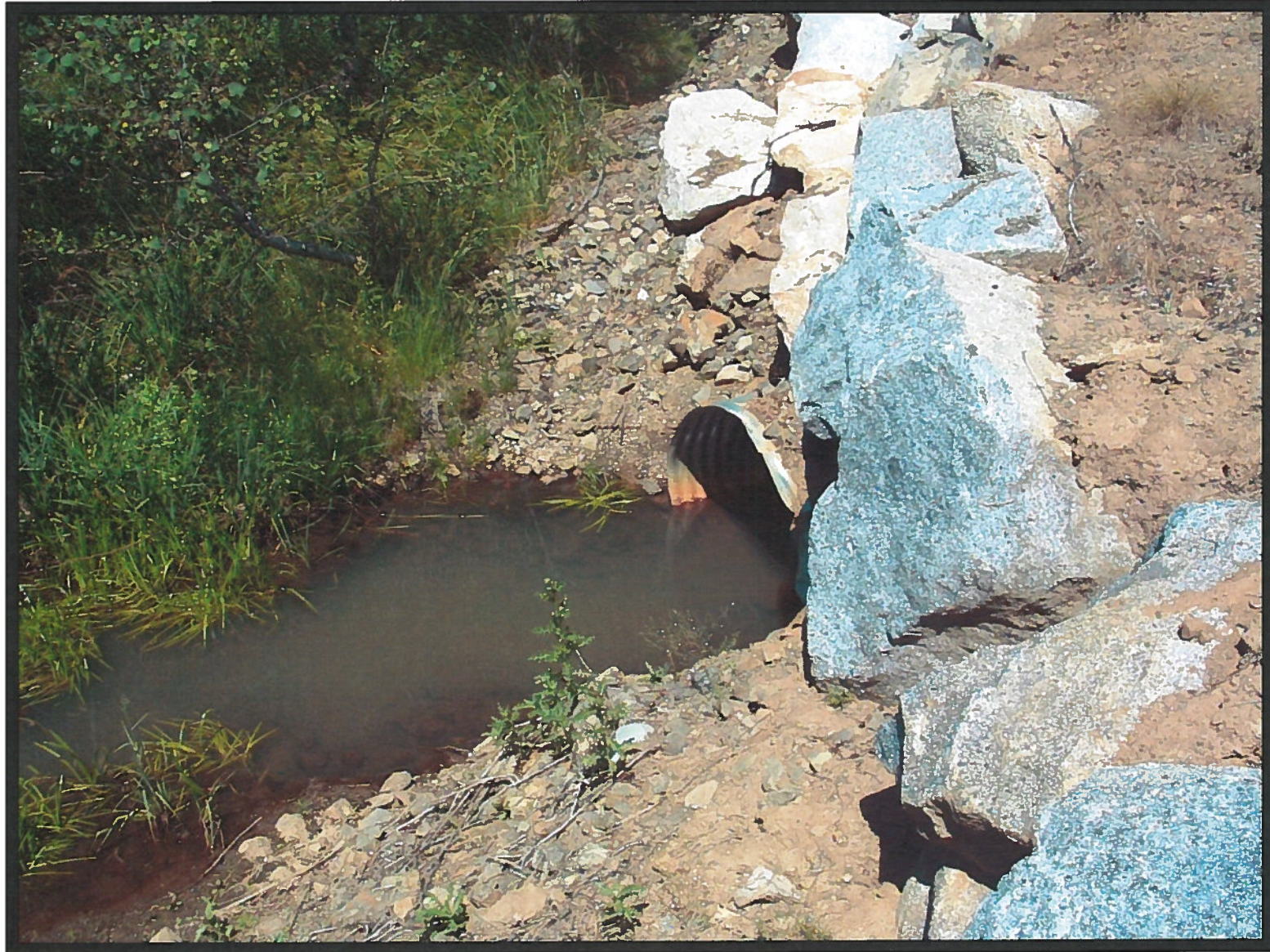
Unnamed Stream Bypass Culvert Outlet
