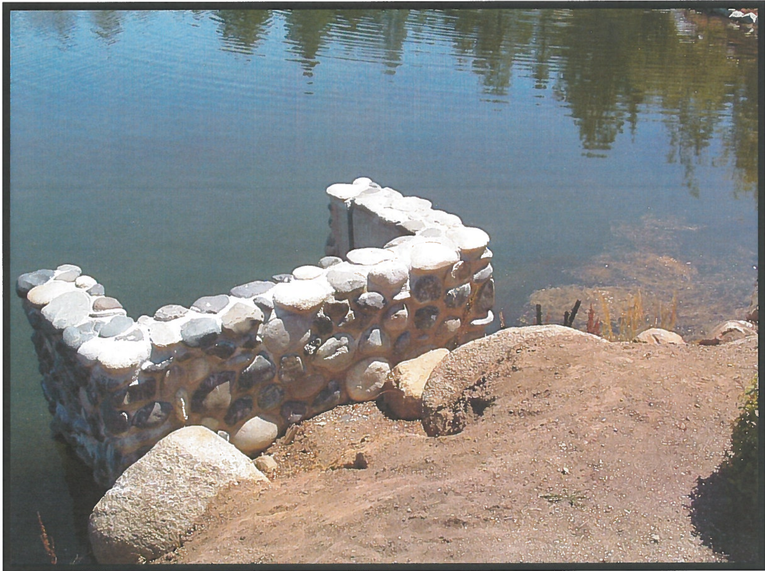
Betsy Pond Overflow to Recirculation Pump
