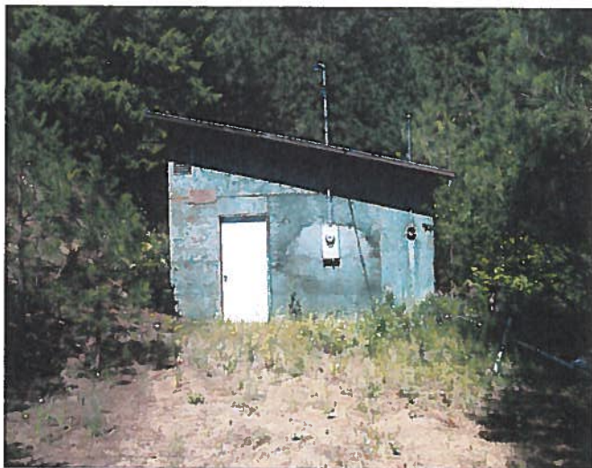
Figure 2-2: Existing Wood-Frame Mechanical Room
