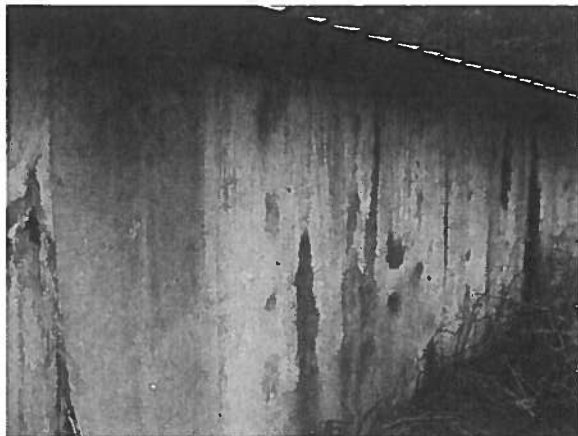
Figure 2-1: Existing Concrete Reservoir with Wood Rafters
