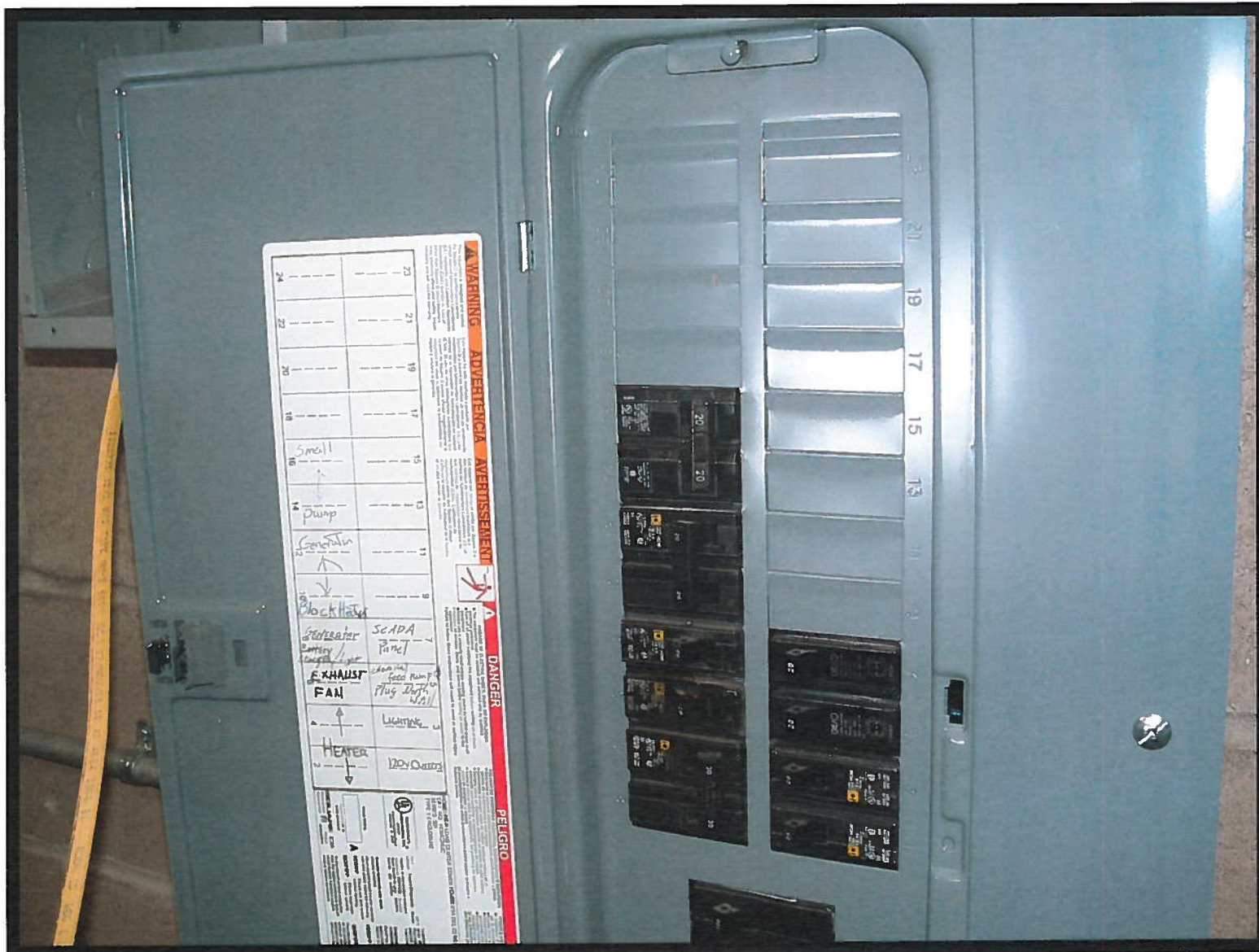
1-hp pump breaker
