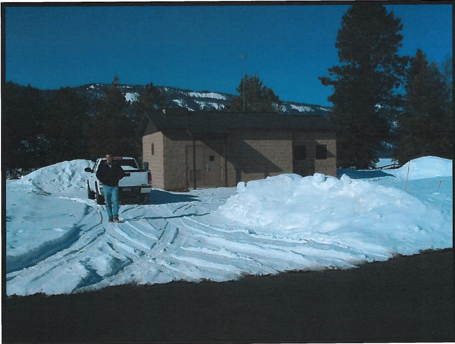
Well house – view from street
