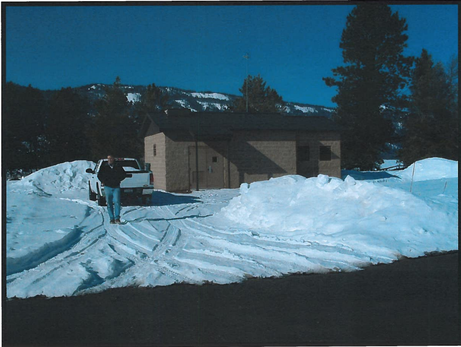
Well house – view from street
