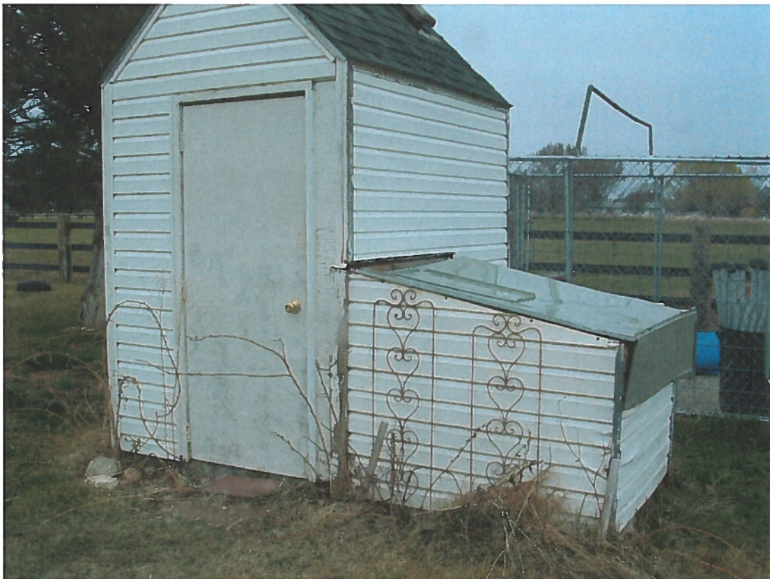
Well house (left) and well shelter (right)
