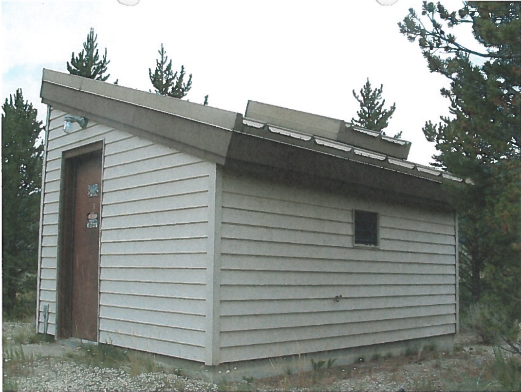
Well 3 well house
