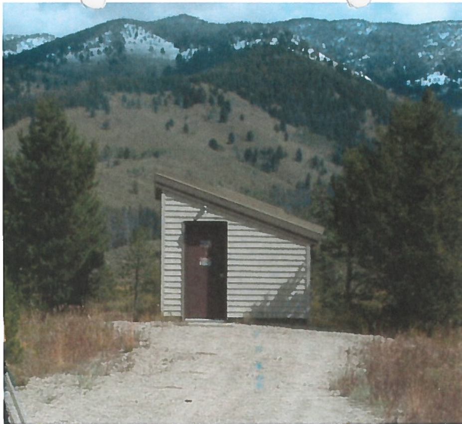
Well 1 well house
