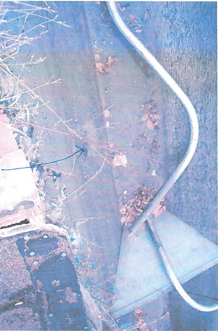
PIC#2 Cement ditch with inlet from pump
