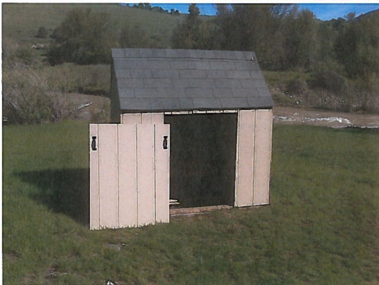
Pump Control Building
