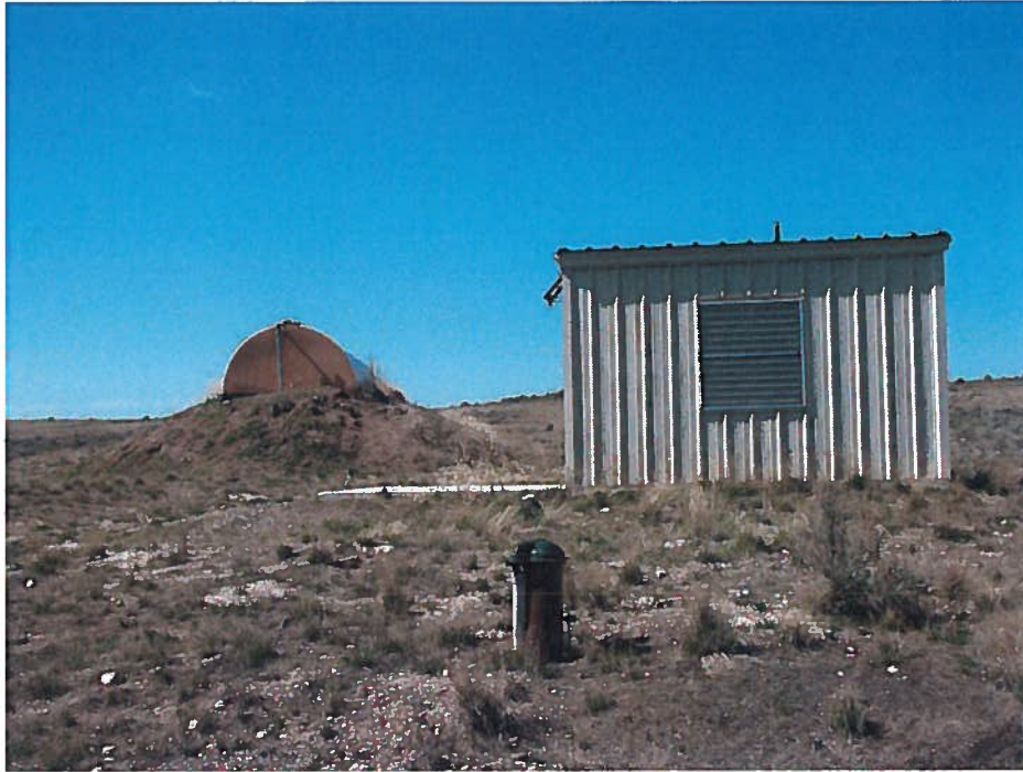
Figure 1: Well Head, Pump House and Storage Tank.
