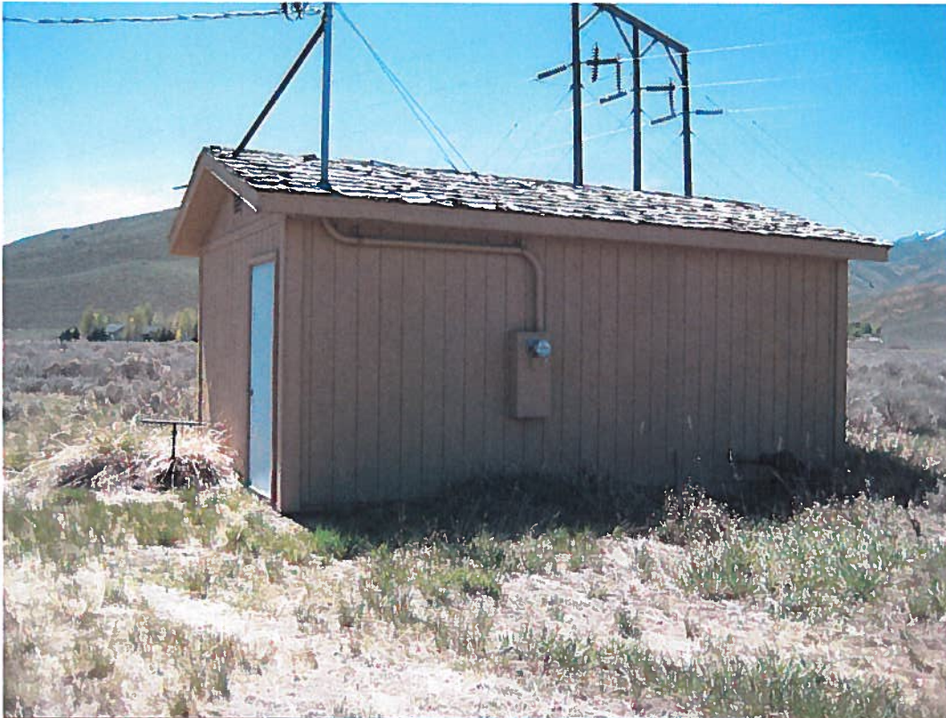
well house looking NW
