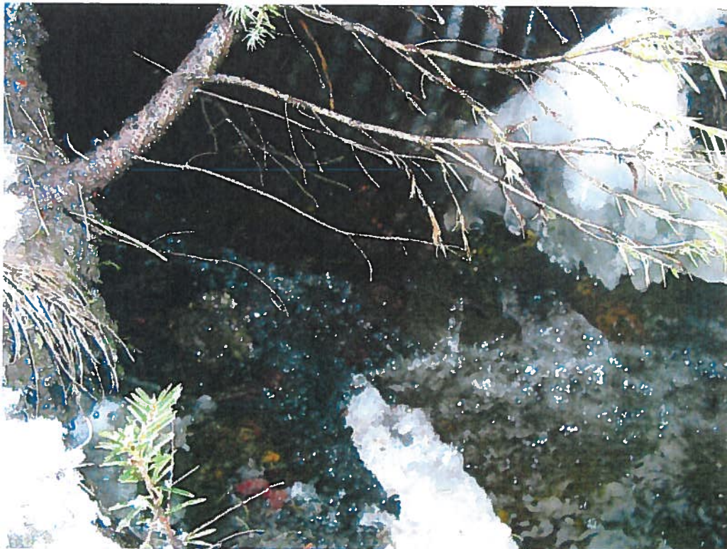
JR Allen Site Visit 11/17/2011 Photo #2: Unnamed Stream (Richard's Creek) culvert underneath West Mountain Rd, downstream side.
