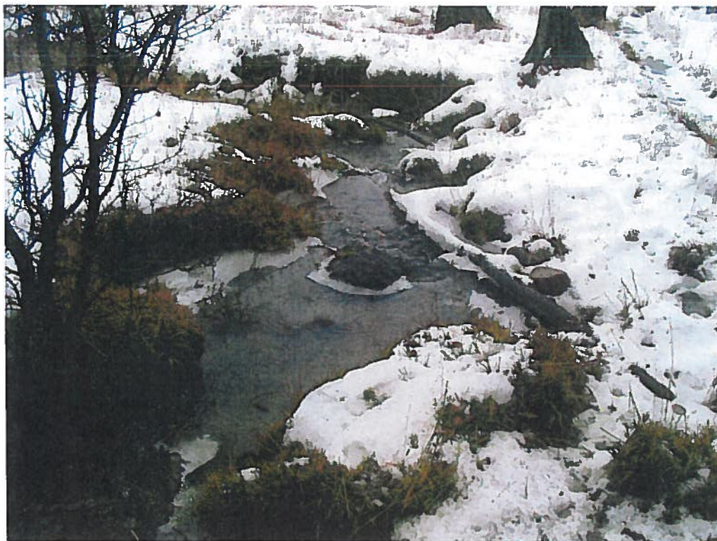
JR Allen Site Visit 11/17/2011 Photo #5: Allen Ditch inside pasture, approximately 5 ft downstream of culvert.
