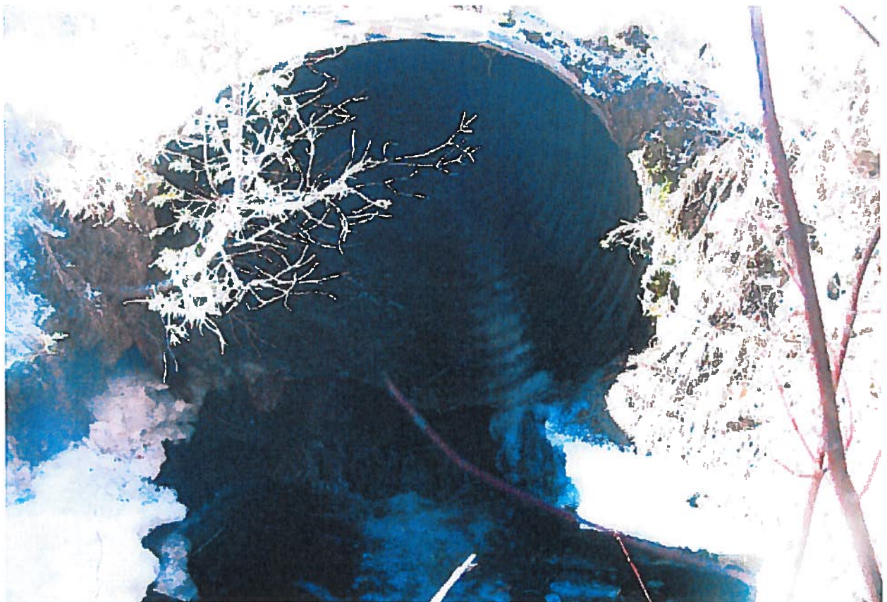
4. Richards/Rock Creek culvert under W. Mtn. Road. Flow is still open, thin ice over the top.
