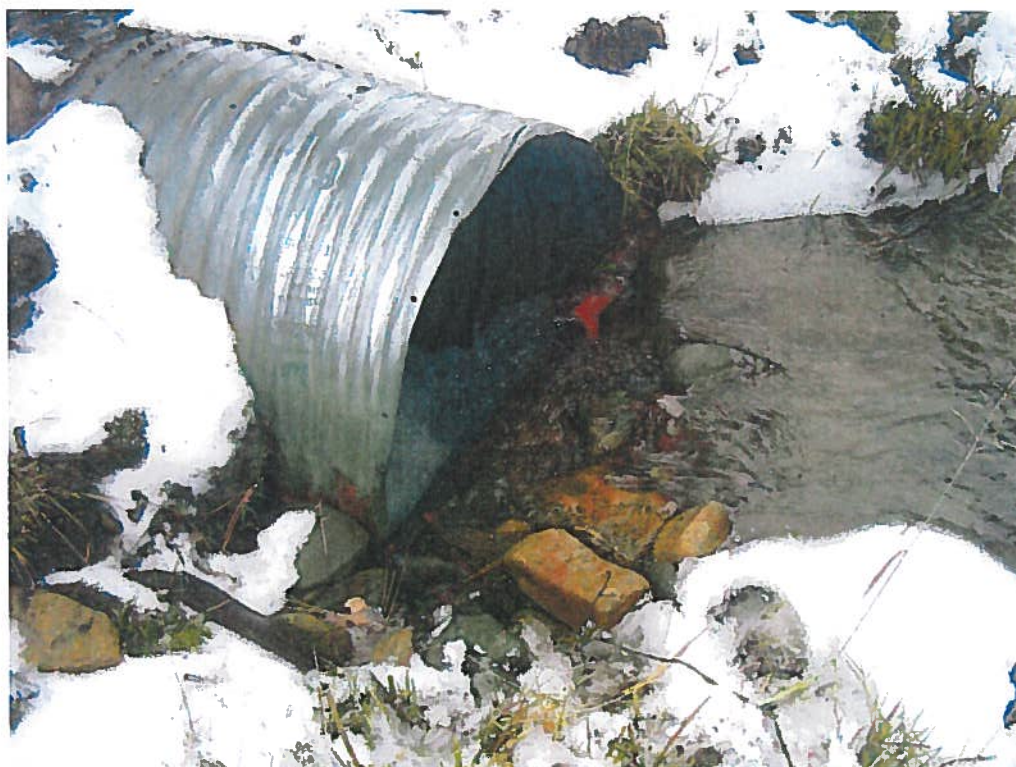
JR Allen Site Visit 11/17/2011 Photo #4: Allen Ditch culvert inside pasture, upstream side.
