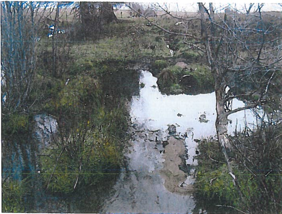
Chess/JR Allen Complaint 11/18/2010 Photo #2: POD for southside acres of right 65-3111X. Water diverted from Rock Ck "Richard's Ck" (foreground and far left of picture) via rusted culvert pipe and ditch (middle ground right of picture).
