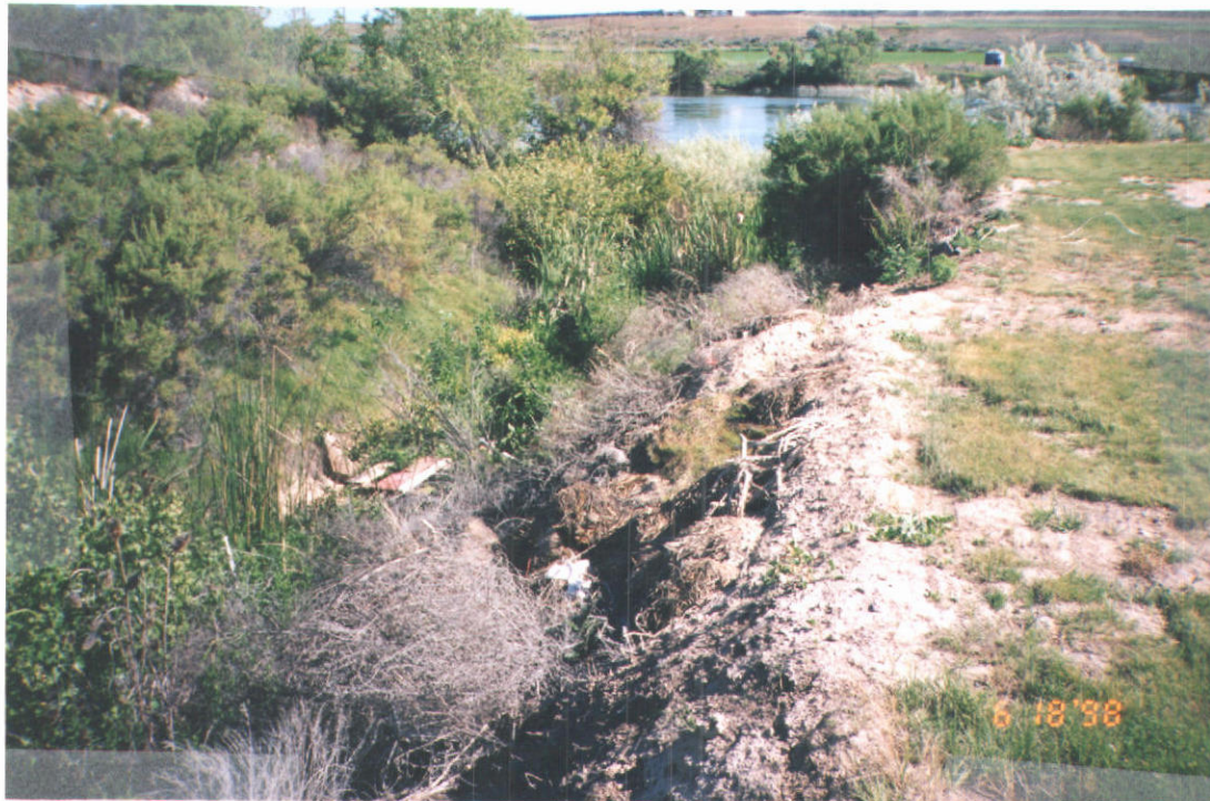
View Looking North (Spill Piles on left)
