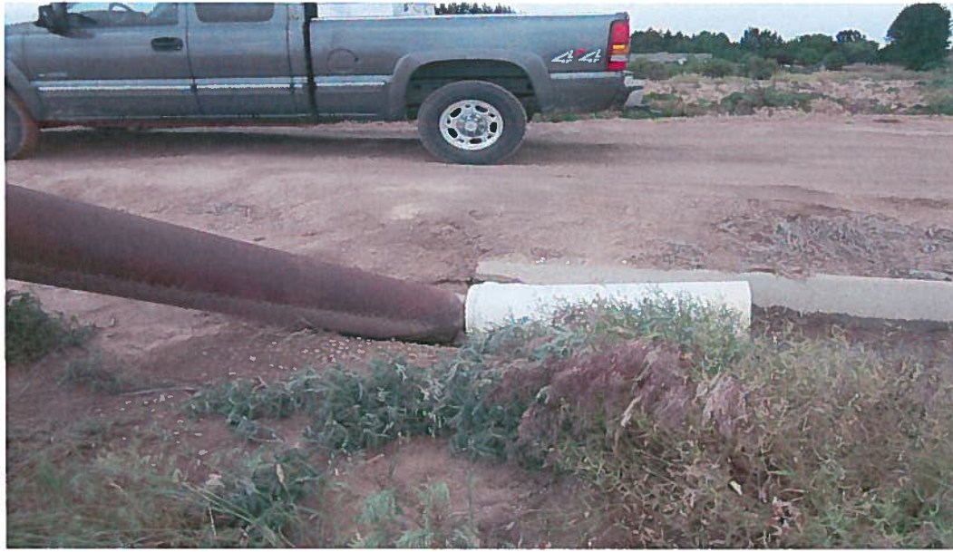
Pipe from corrugated steel collector to open concrete lined ditch.
