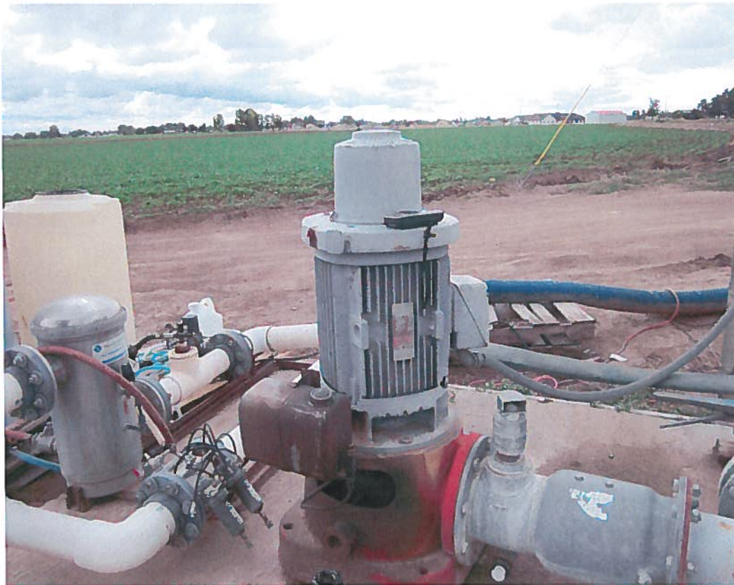
Well. Fertilizer system seen to left. Steel pipe from well seen front right.
