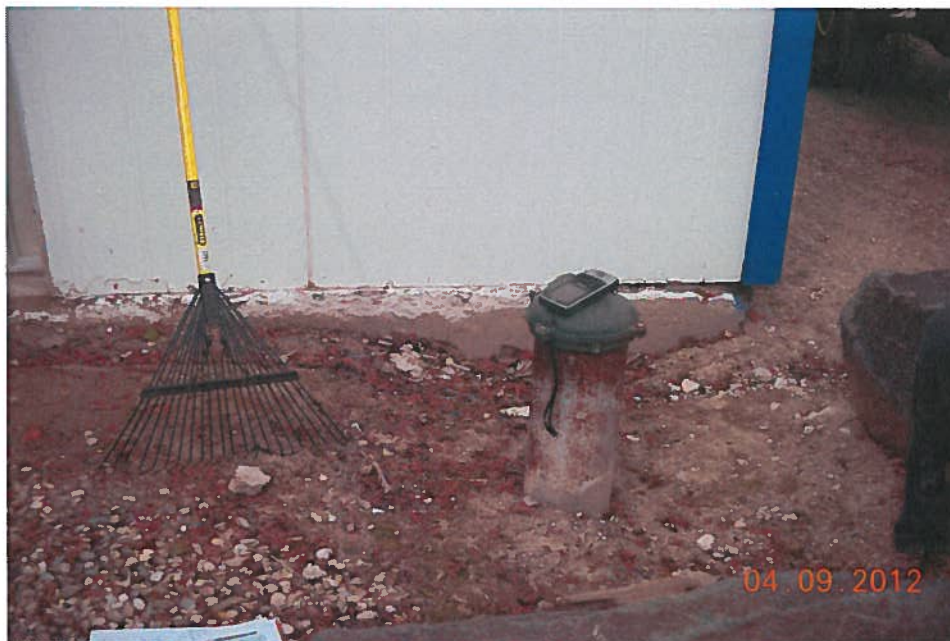
The 6" well drilled in 1975 for the Decoy Inn Drive-In. Used for internal domestic for RVs, irrigation of the 0.009 acre yards + common area, the laudromat and the studio. Well is about 2' east of the large shed on the south property line
