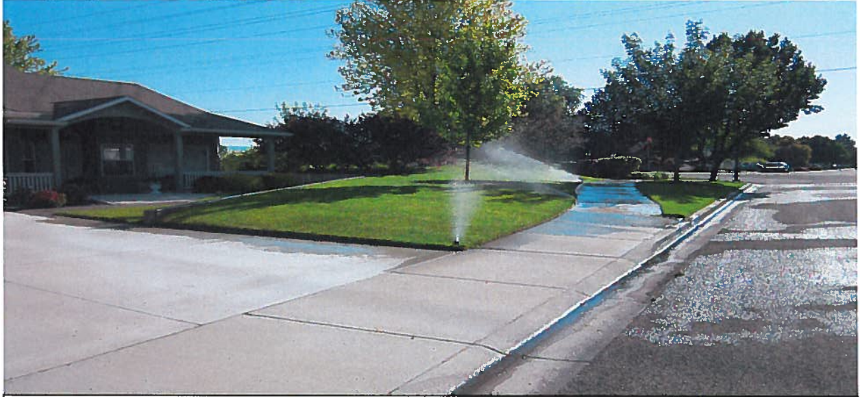
Place of use. View northeast of typical pop-up sprinkler system within residential lots.
